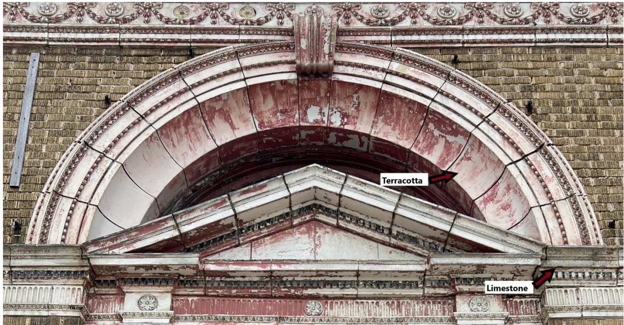
Figure 10: Detail view of the west volume's arched window, calling out the subtle difference in appearance between the terracotta and limestone ornamentation, divided by the stringcourse.
