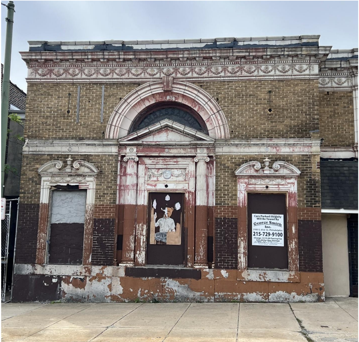
Figure 9: View of the facade's east volume.
