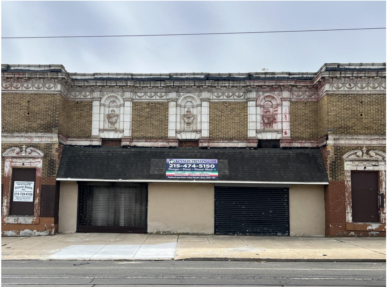
Figure 11: View of the facade's central volume.
