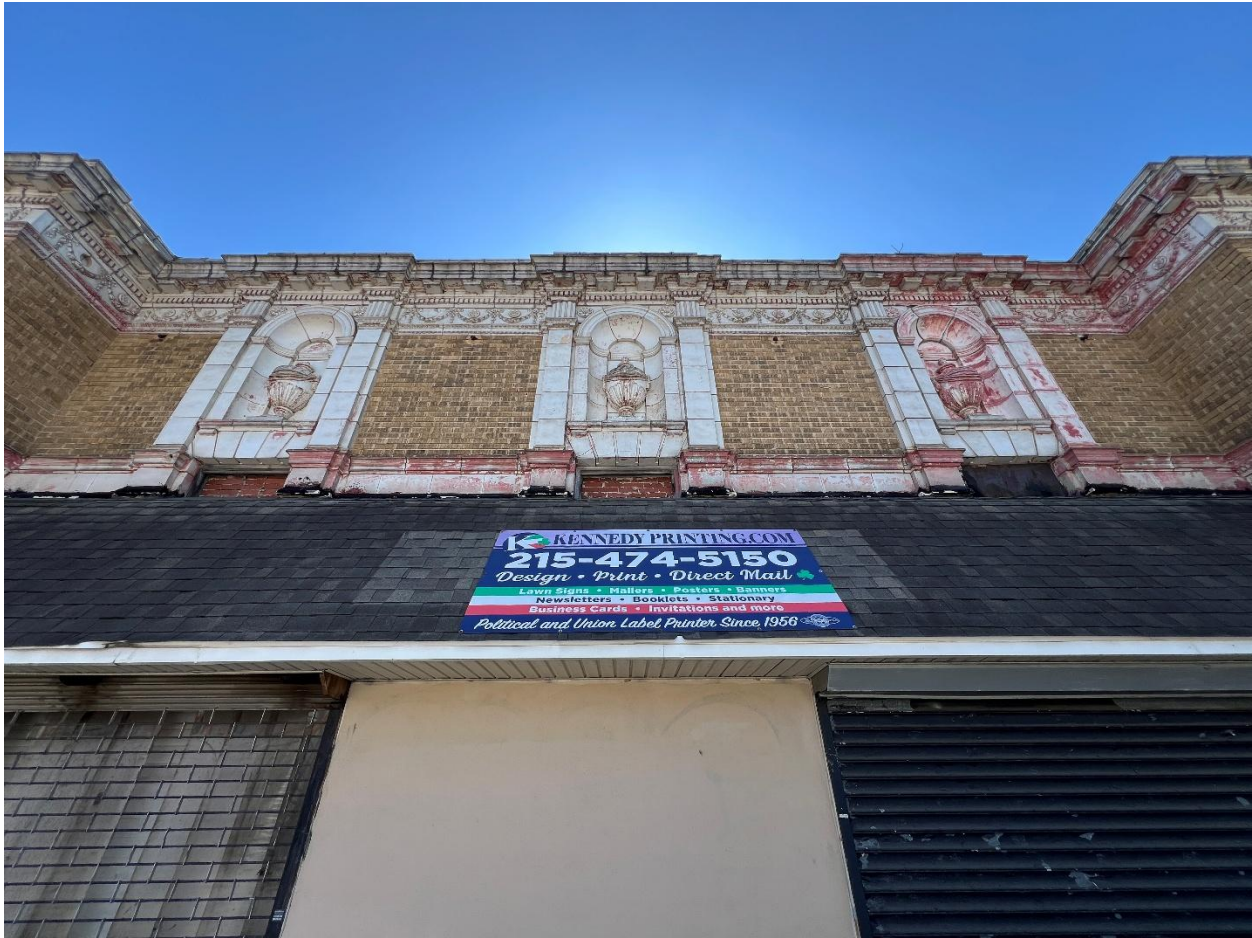
Figure 12: View of the facade's central volume.
