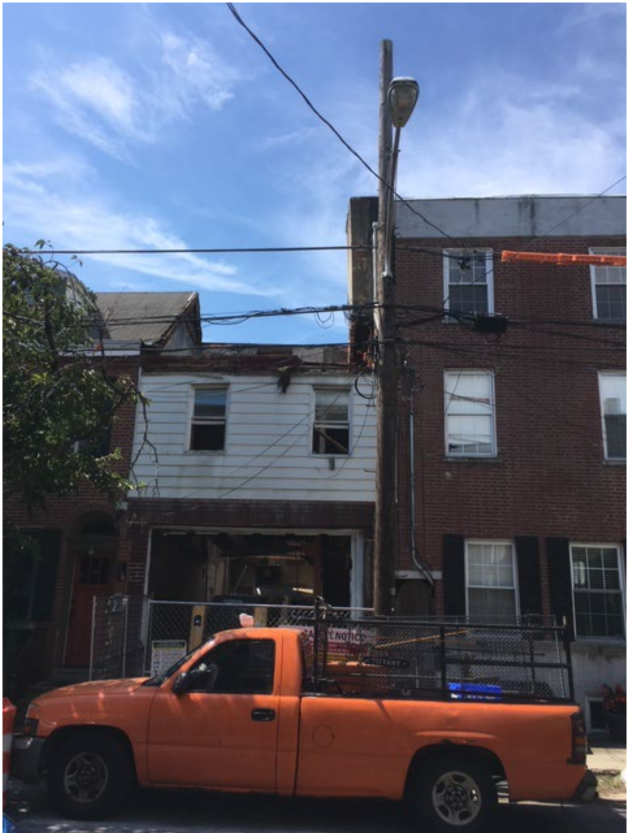
Figure 4. Demolition in progress, July 20, 2020.
