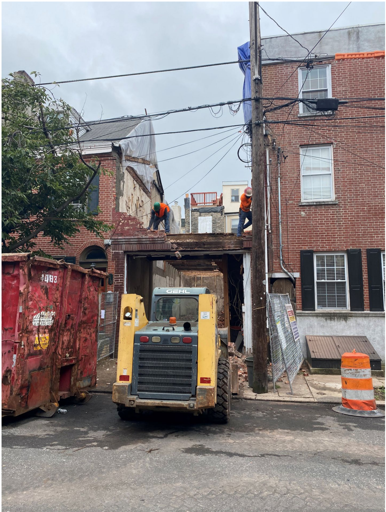
Figure 5. Demolition in progress, July 23, 2020.
