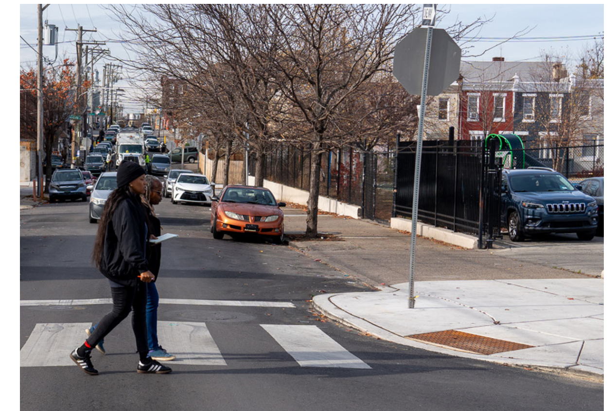
Above: Concrete curb extension in the Cramp Slow Zone.
