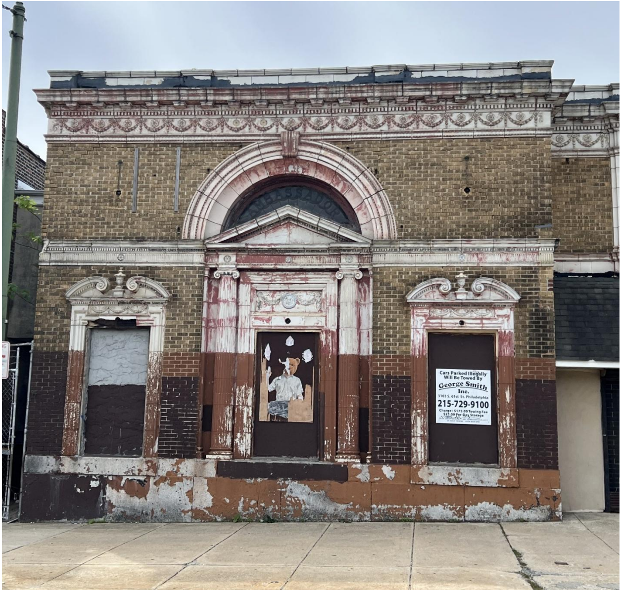
Figure 9: View of the facade's east volume.
