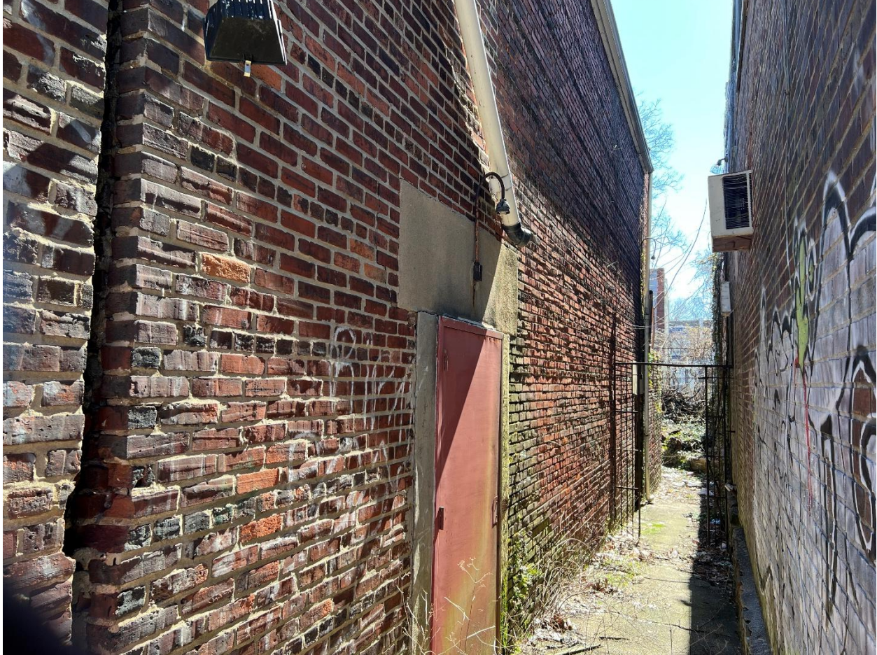
Figure 22: View of the Ambassador Theatre's west elevation.
