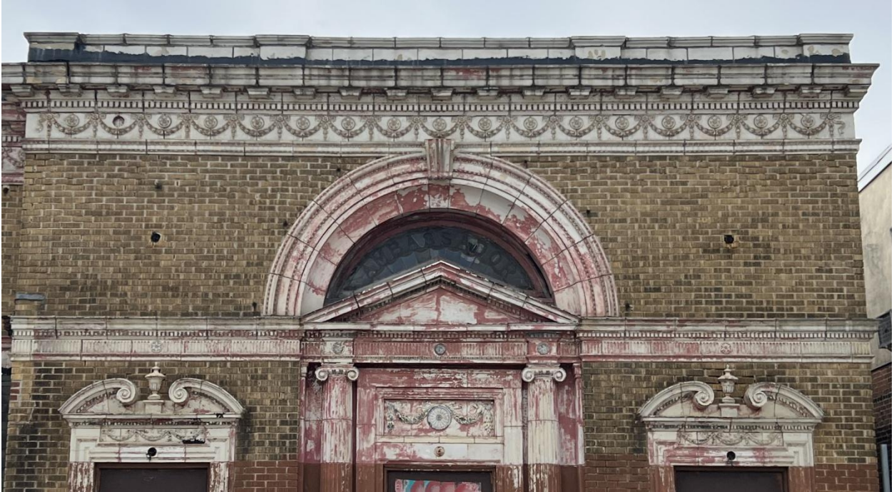
Figure 17: Detail view of the upper level of the facade's west volume.
