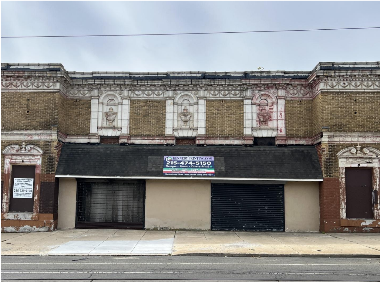
Figure 11: View of the facade's central volume.
