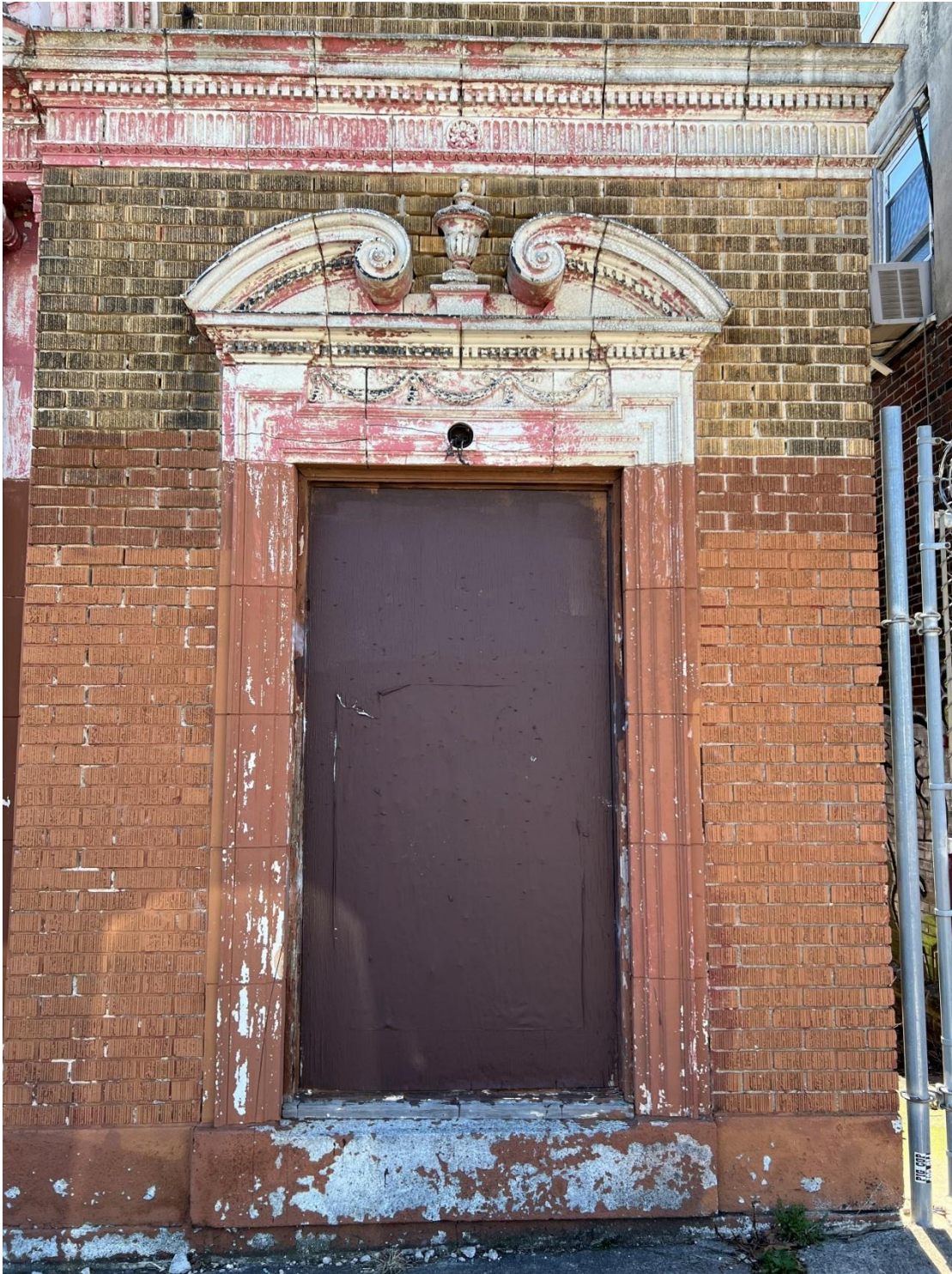
Figure 19: View of the westernmost display board of the facade.
