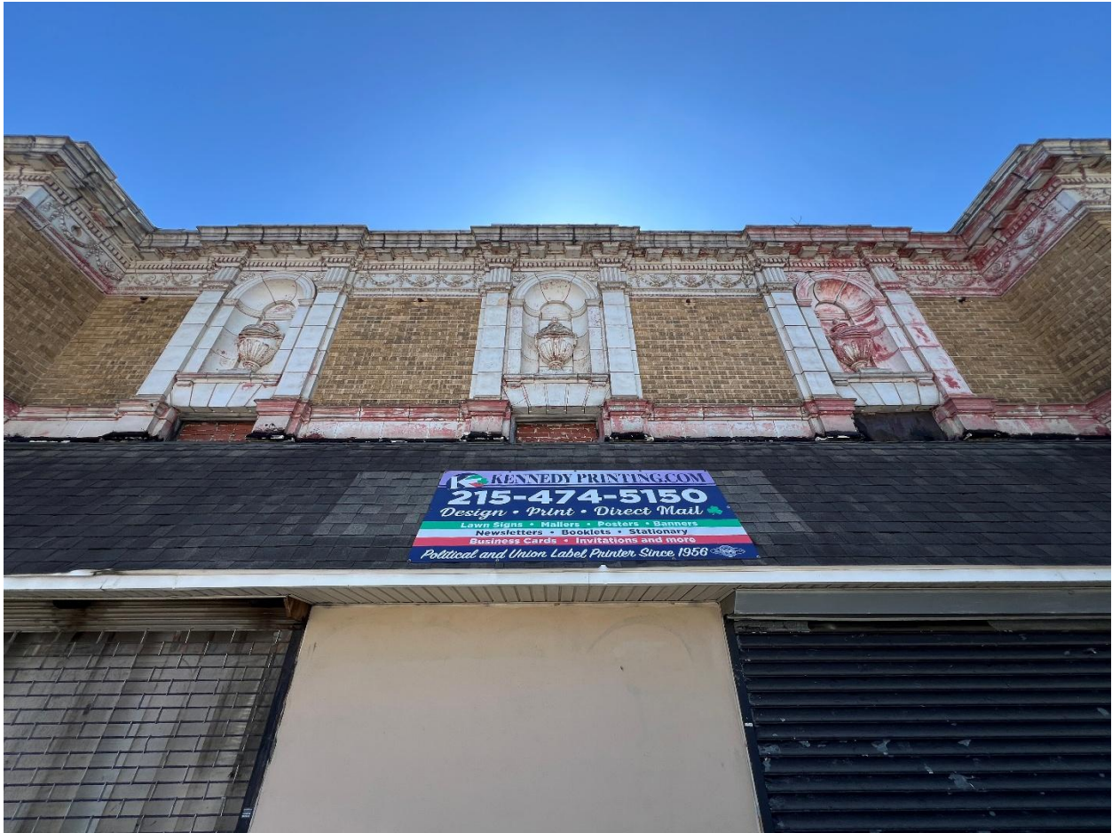
Figure 12: View of the facade's central volume.
