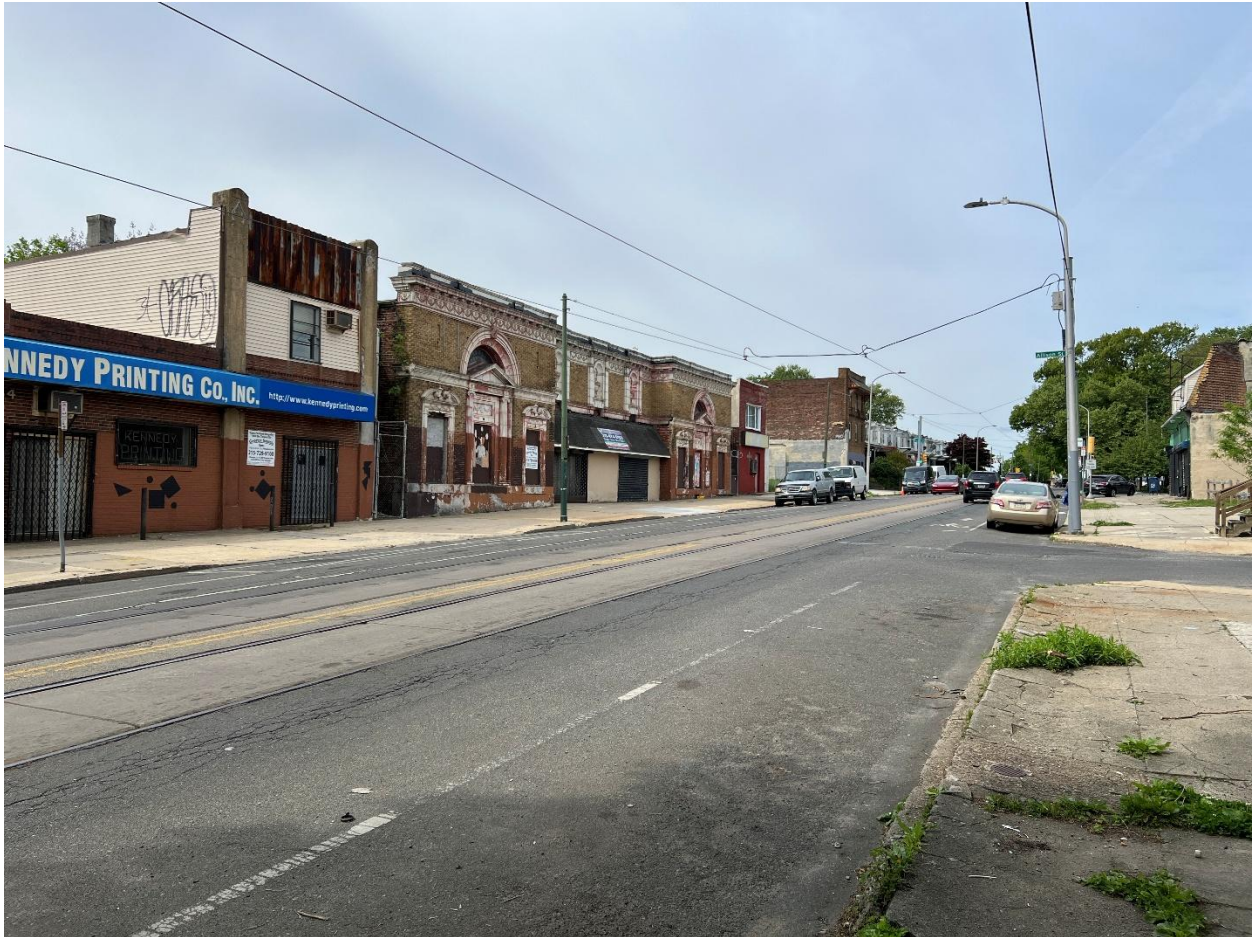
Figure 5: View of the Ambassador Theatre in the context of Baltimore Avenue.
