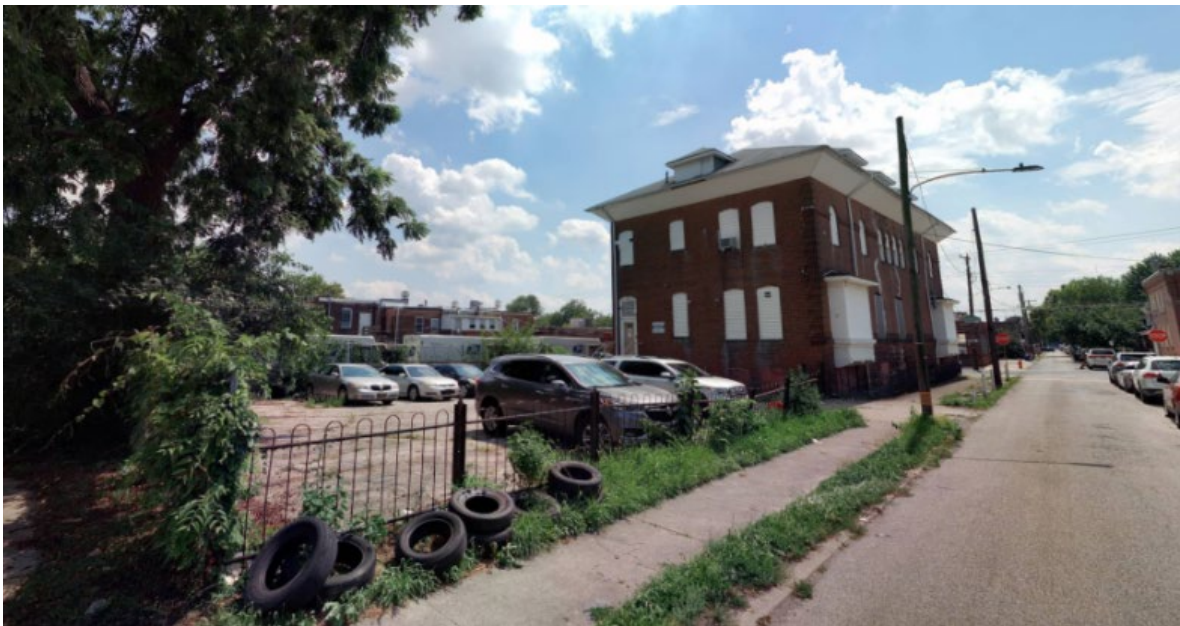
Figure 4: View from Marsden St (facing southwest) of rear of subject property.
