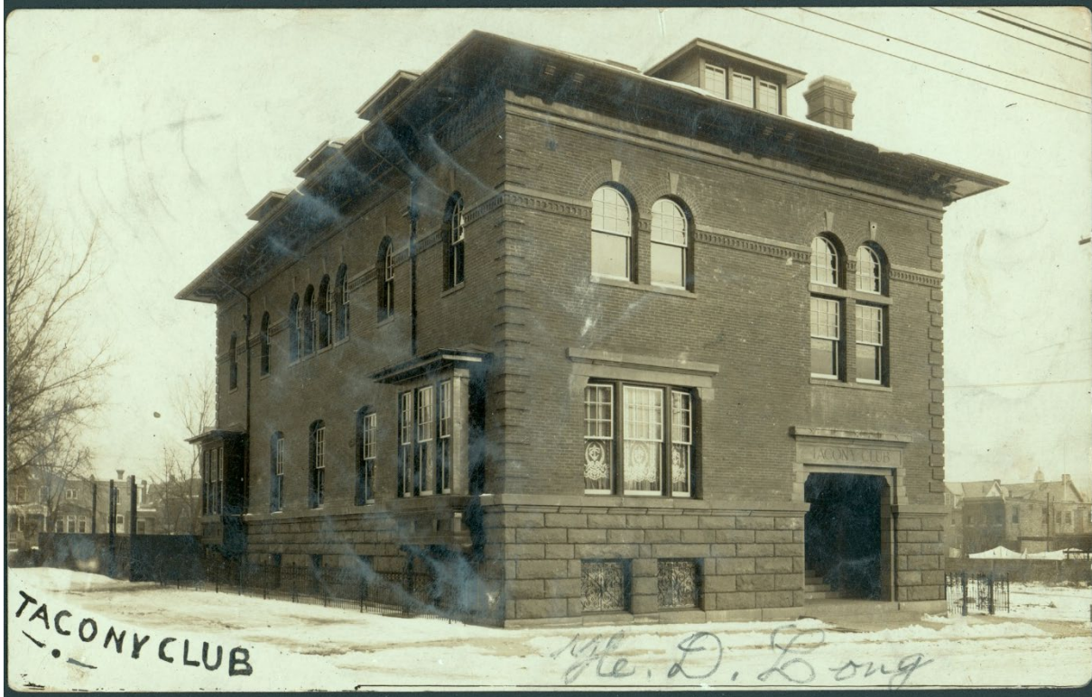
Figure 7: Early photograph (facing east) of the subject property's primary elevations.
