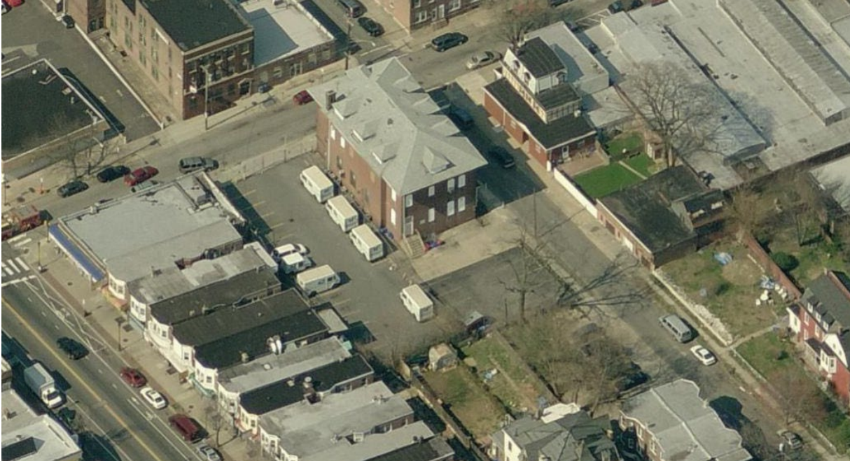
Figure 3: Aerial view (facing west) of the rear of subject property.
