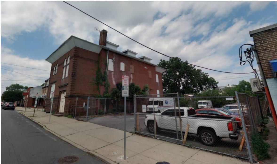
Figure 8: View from Longshore Ave (facing north).
