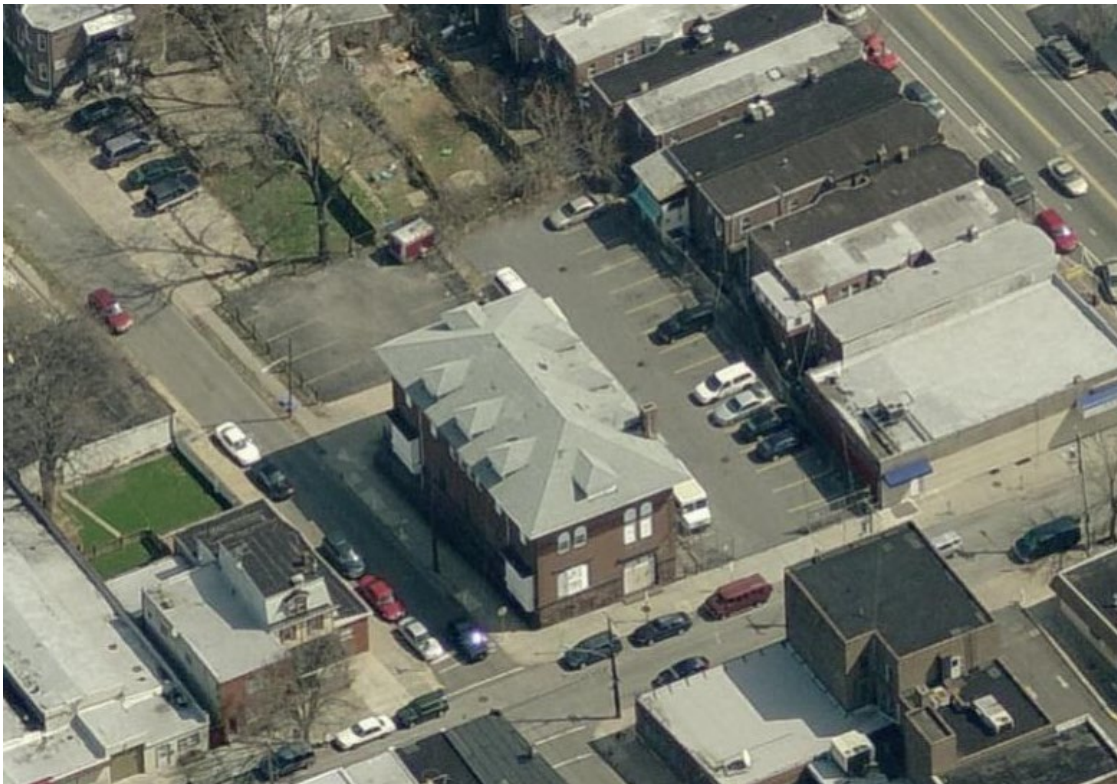
Figure 2: Aerial view (facing east) of subject property's primary elevations along Longshore Ave and Marsden St.
