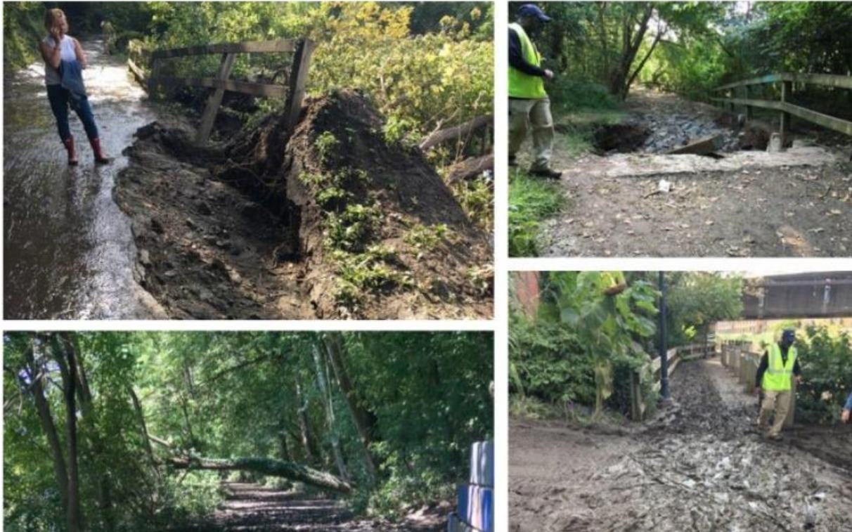
Figure 4: Impacted Trails and Parks Infrastructure
