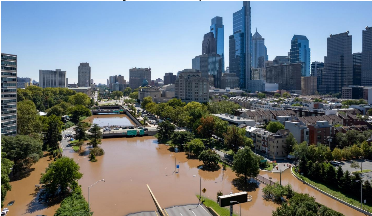
Figure 12: Interstate 676 after Hurricane Ida
