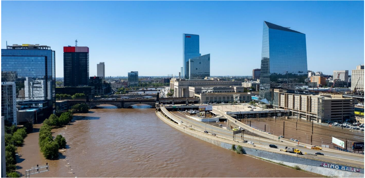
Figure 13: Interstate 676 after Hurricane Ida
