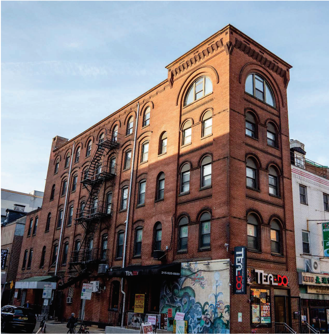
Figure 1. The south and east elevations of 132 N. 10 th St. Image courtesy of nominator
