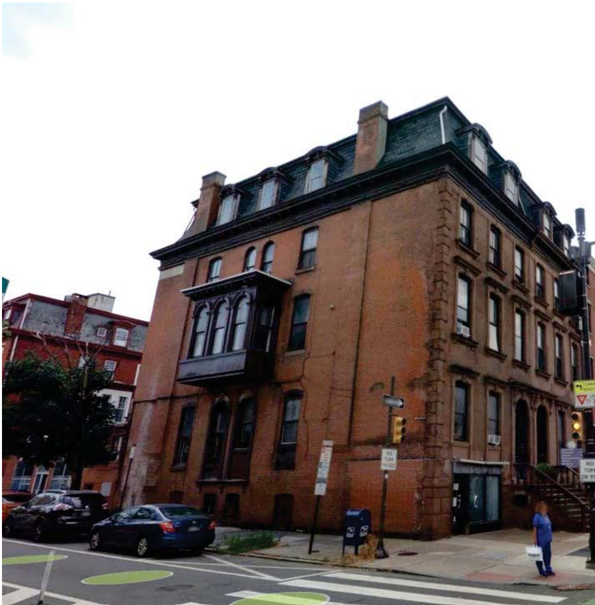
Figure 3: 1000 Spruce St., Side Facade. July 2025. Source: Cyclomedia.
