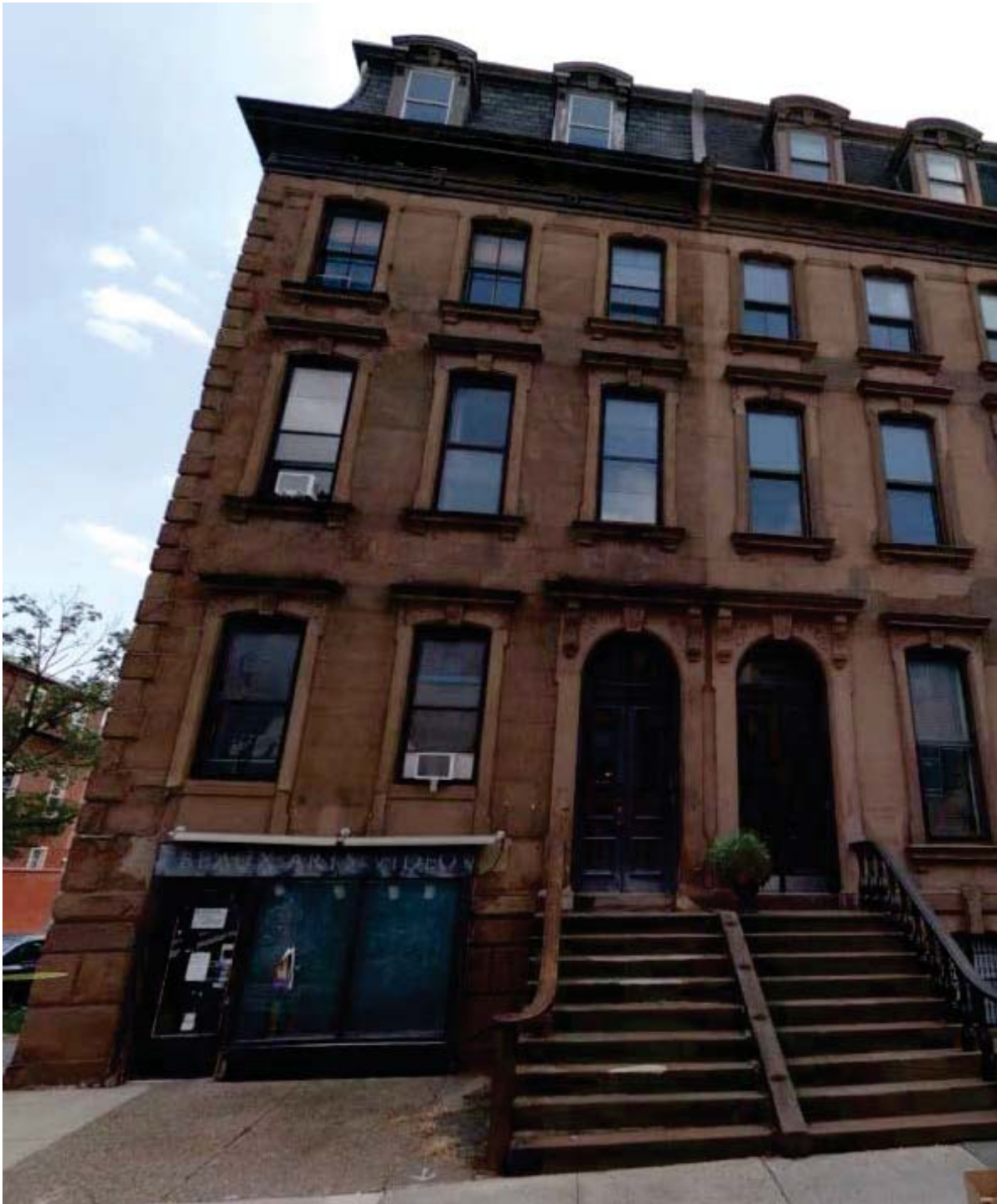
Figure 2: 1000 Spruce St., Front Façade. July 2025. Source: Cyclomedia.
