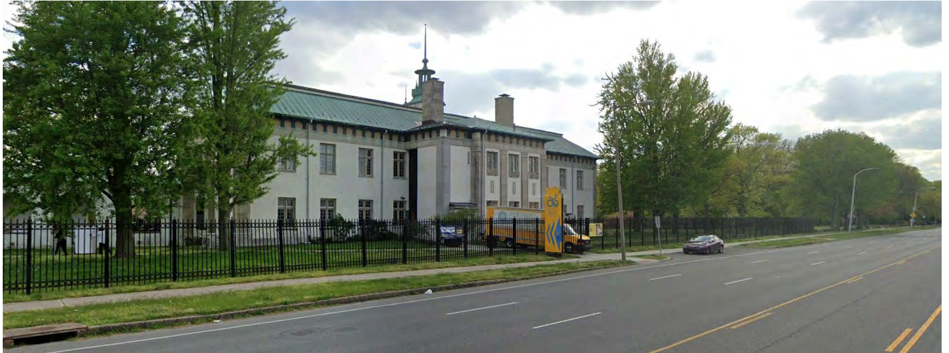
SITE APPROACH- PATTISON AVE
