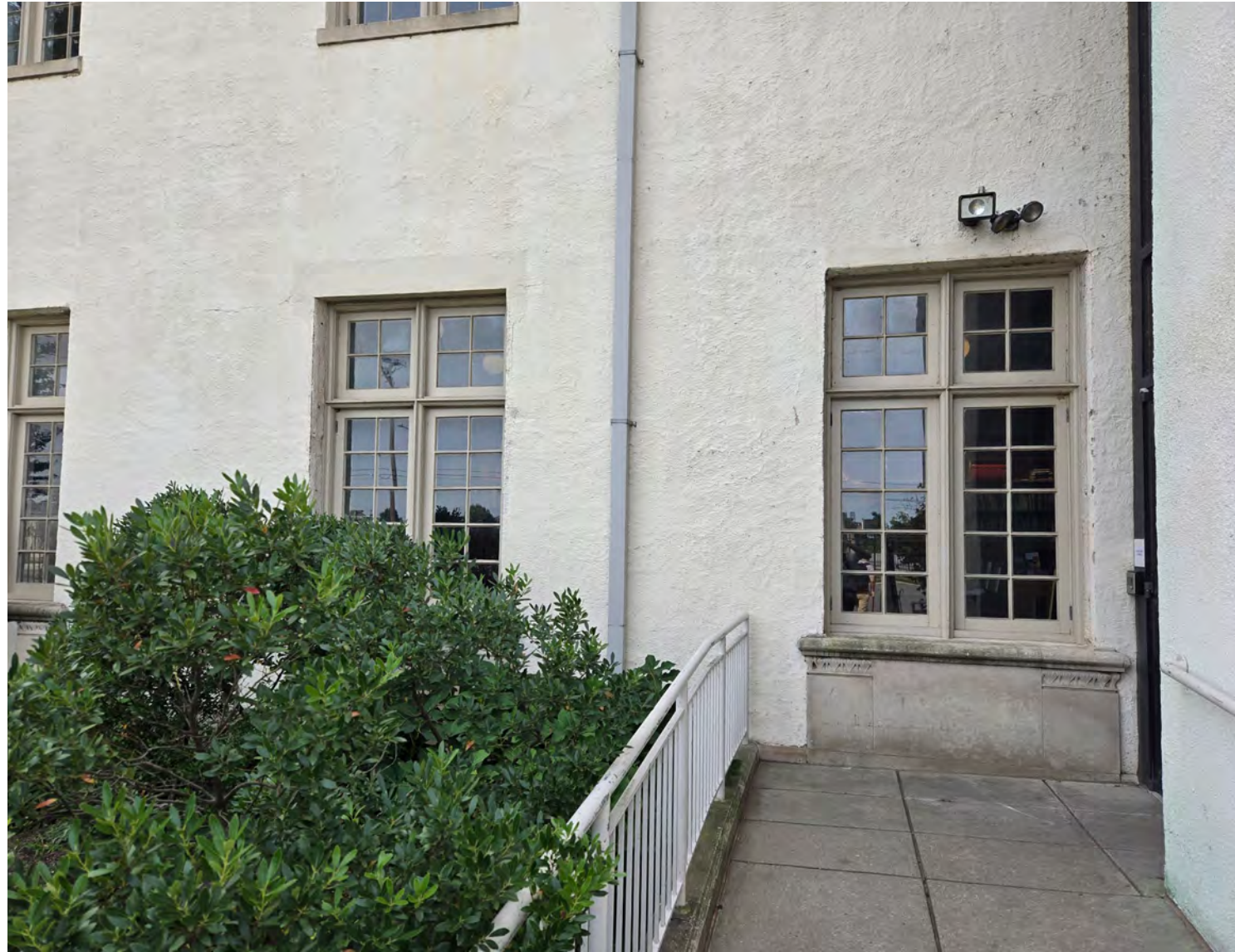
PATTISON AVE BUILDING ENTRY AND ACCESSIBLE RAMP
