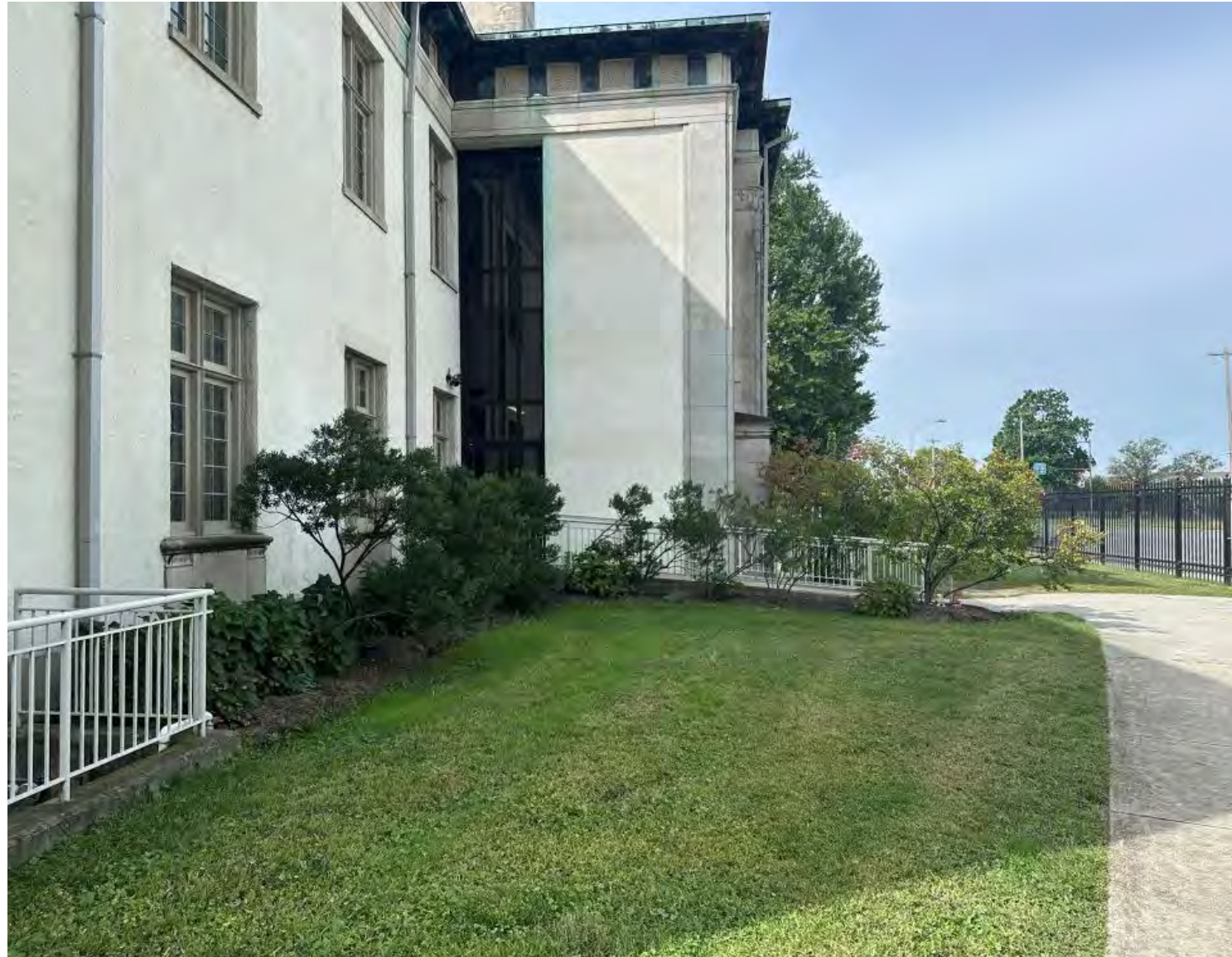
PATTISON AVE BUILDING ENTRY AND EXISTING WALKWAY
