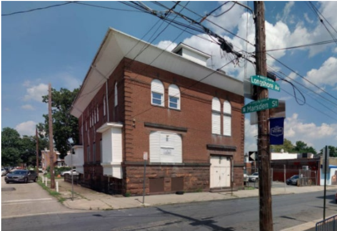
Figure 6: View (facing east) of the subject property's primary elevations.
