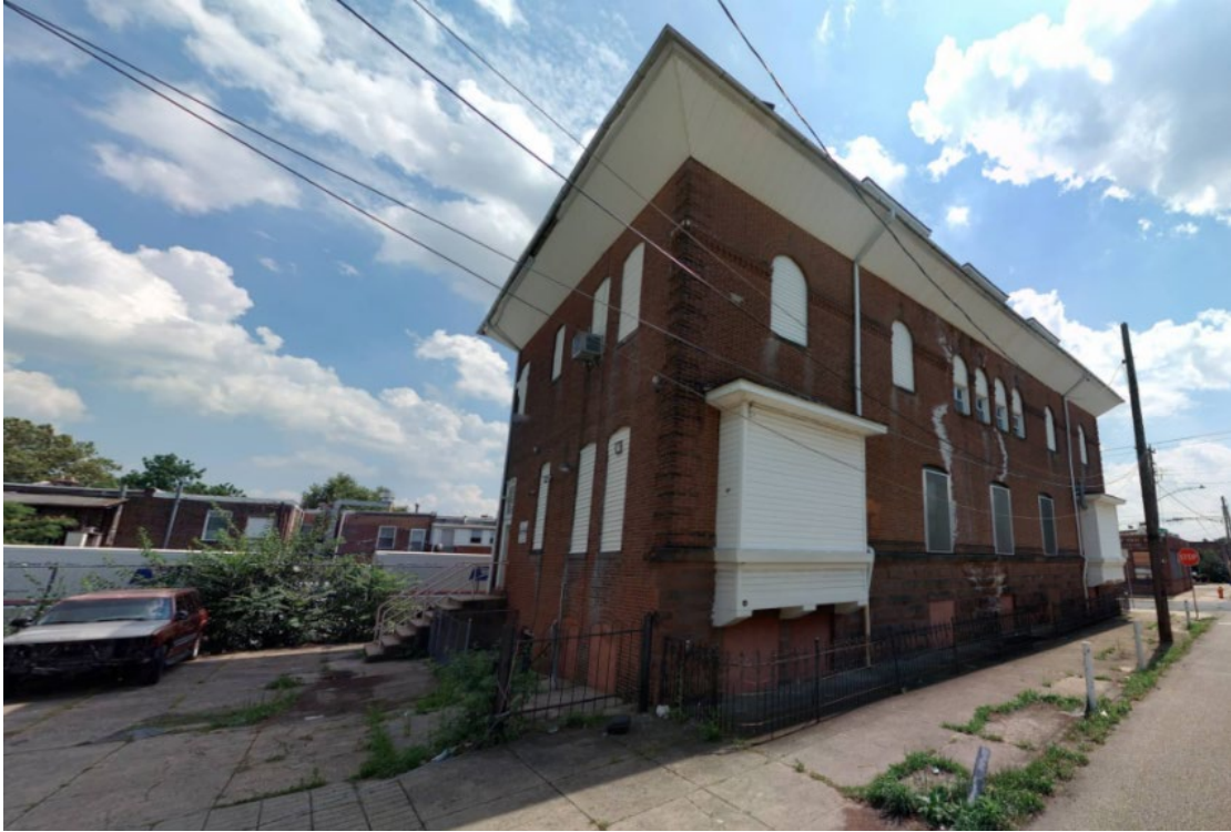
Figure 5: View from Marsden St (facing south) of rear and side elevations.
