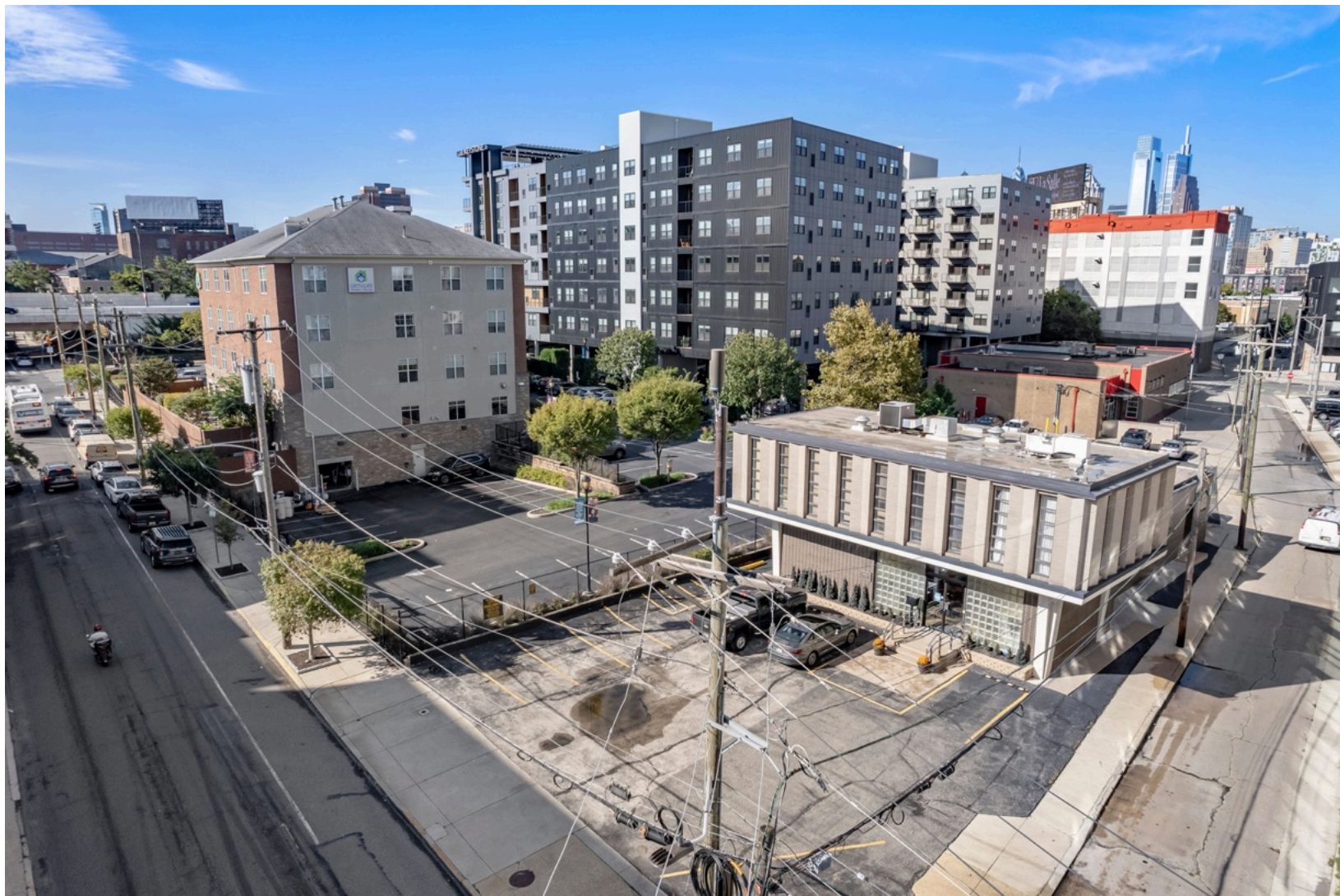
EXISTING SOUTHWEST VIEW
