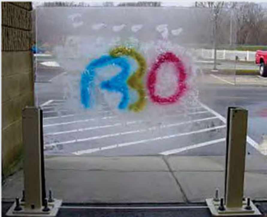
Step 2) Five minutes after remover is applied
