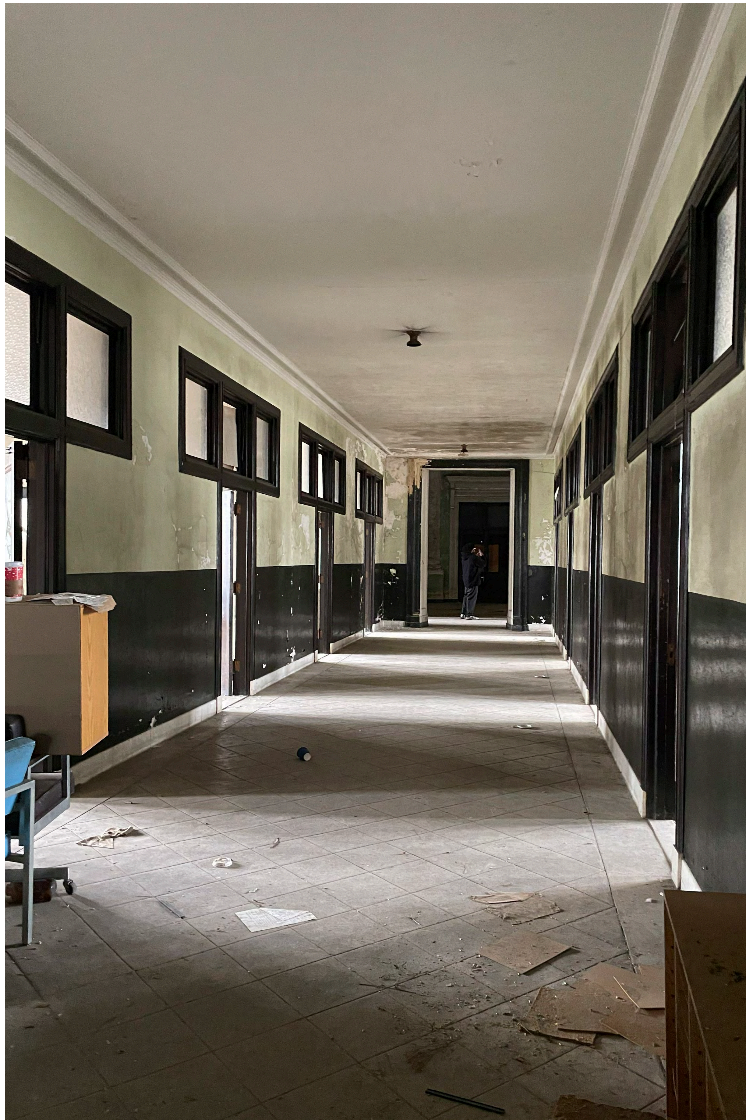
EXISTING - INTERIOR HALLWAY
