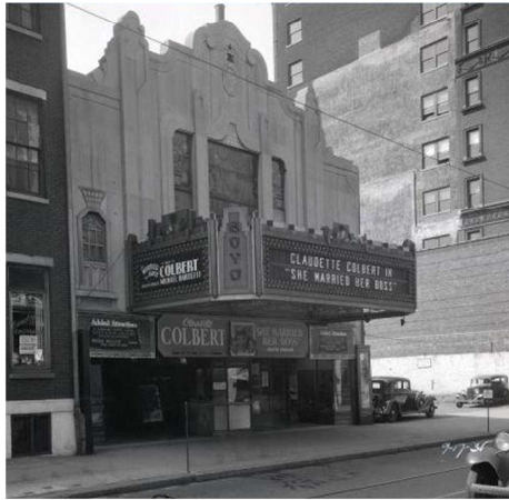
Historical Facade Marquee Condition
