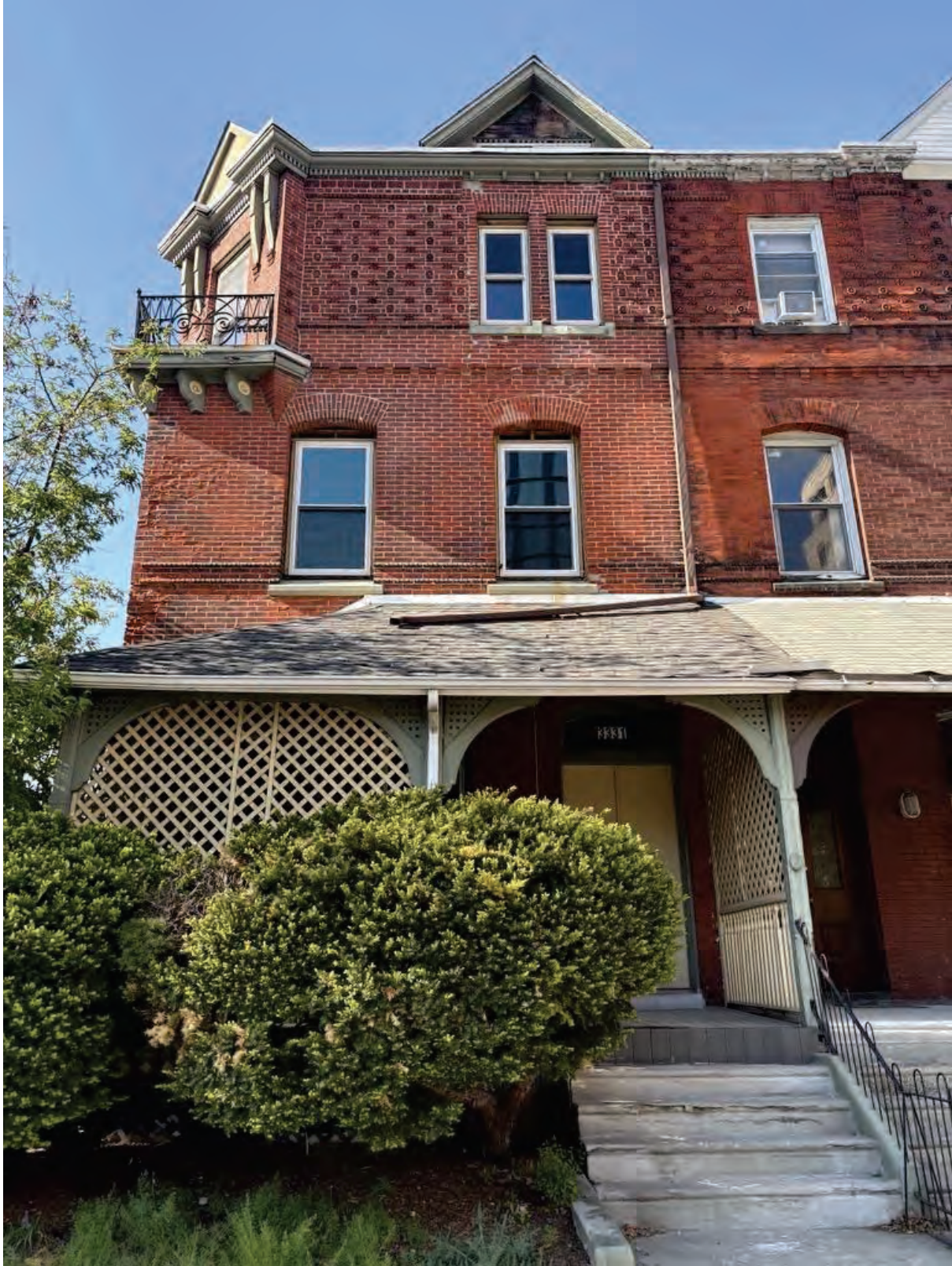
Figure 1. Front façade of 3331 Powelton Avenue with new windows installed. May 2026.
