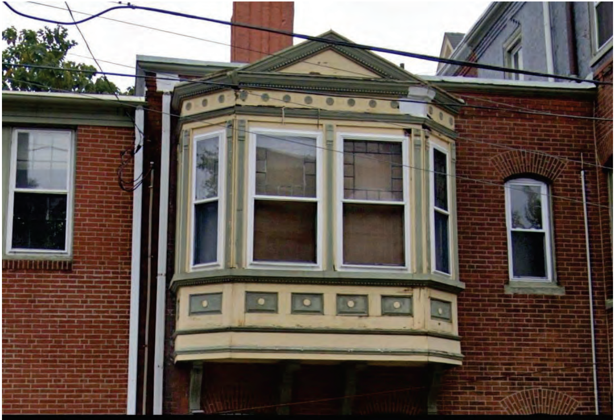
Figure 5. Prior to window replacement. Close up of side elevation bay window with possible original windows in place. October 2024.
