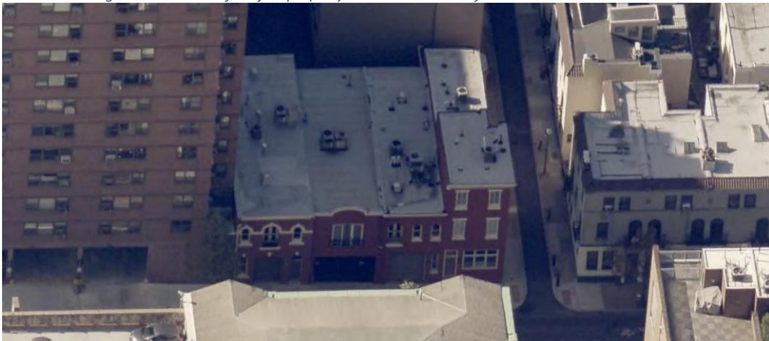
Figure 2: Aerial view of property looking south.
