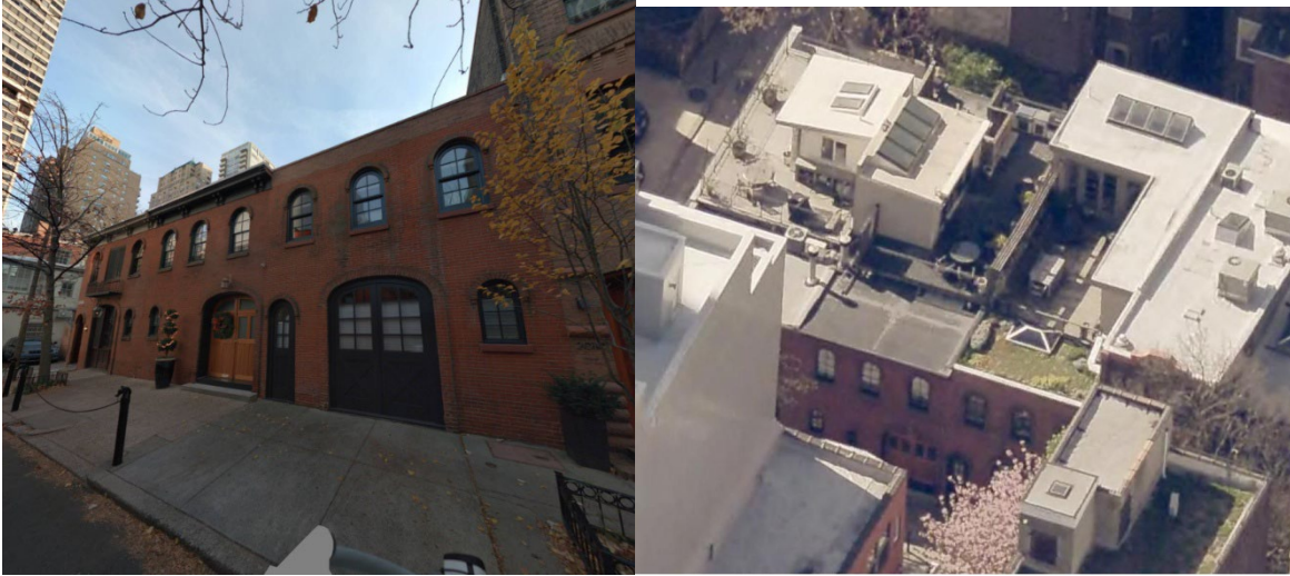
Figure 7: Rooftop additions and decks on (from left to right) 2006, 2008, and 2010-12 Chancellor St were set back to limit visibility from the primary elevation.
