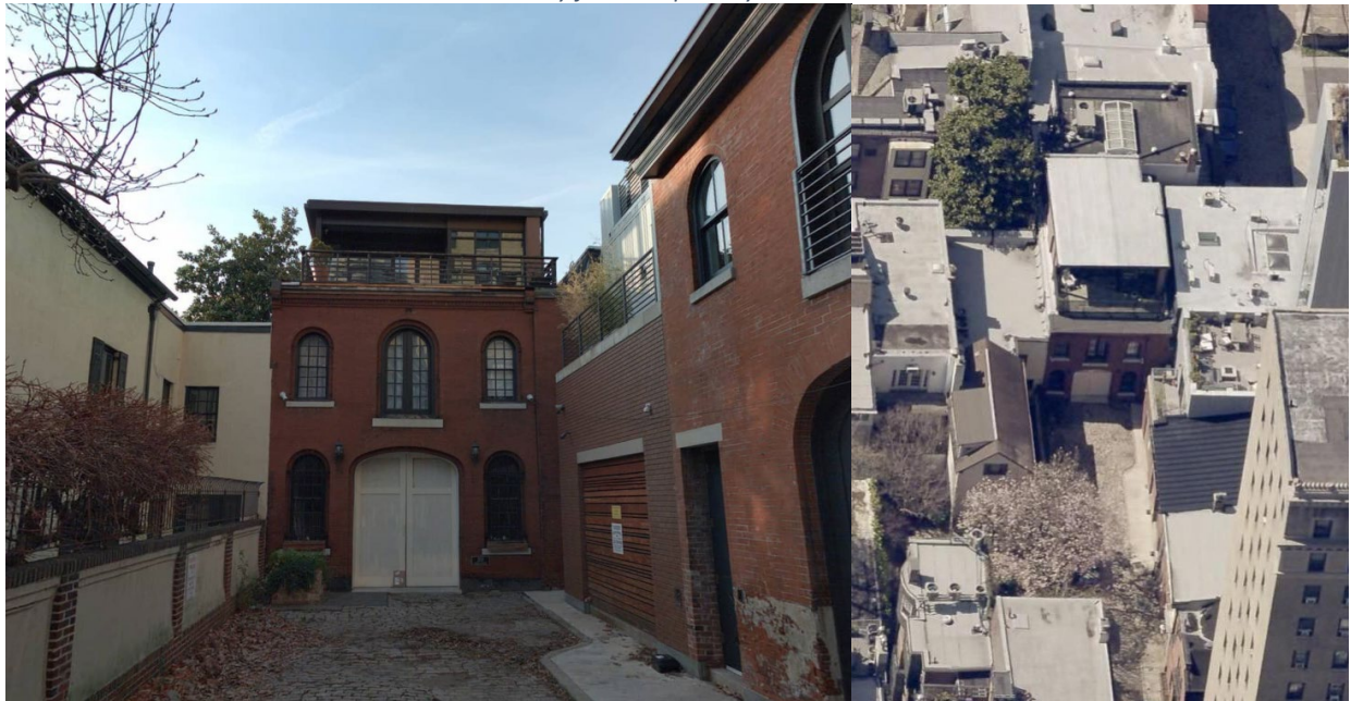
Figure 8: This addition to 2110 Chancellor St, located on a small lot at the dead end of Chancellor St west of S 21 st St, featured contemporary design to differentiate it from the historic building.
