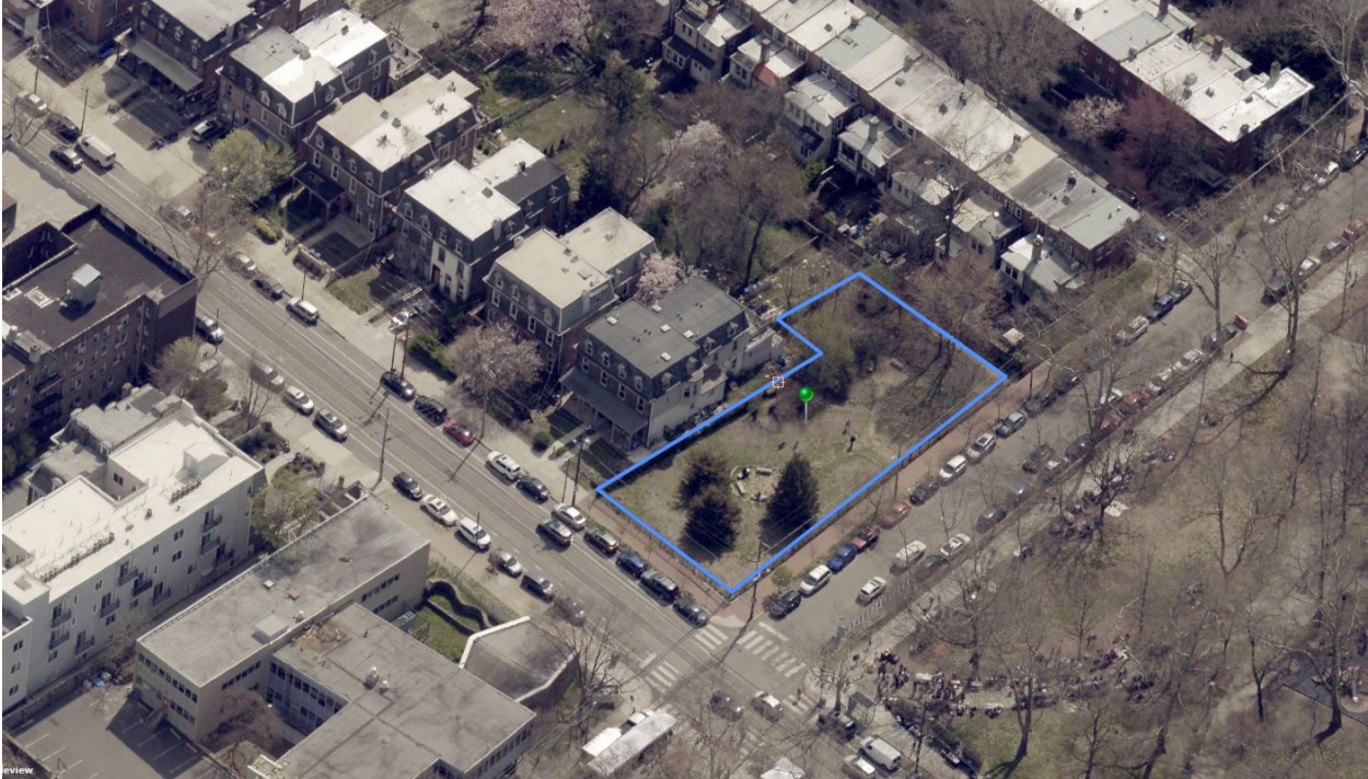
Figure 3: Aerial image of 4238-40 Chester Ave looking SE, Mar 2024
