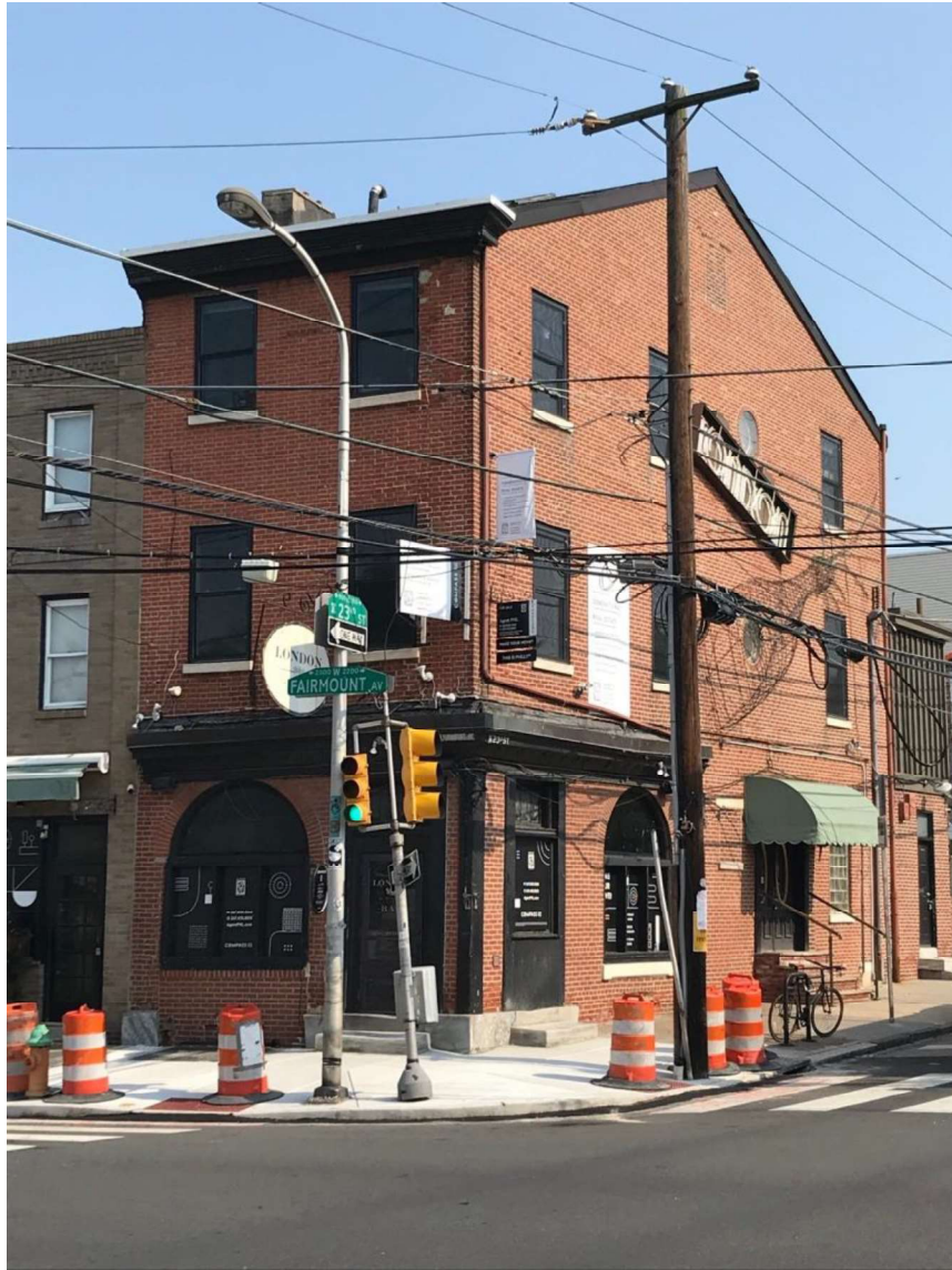
Figure 4 – South and east elevations, looking northwest from Fairmount Avenue.
