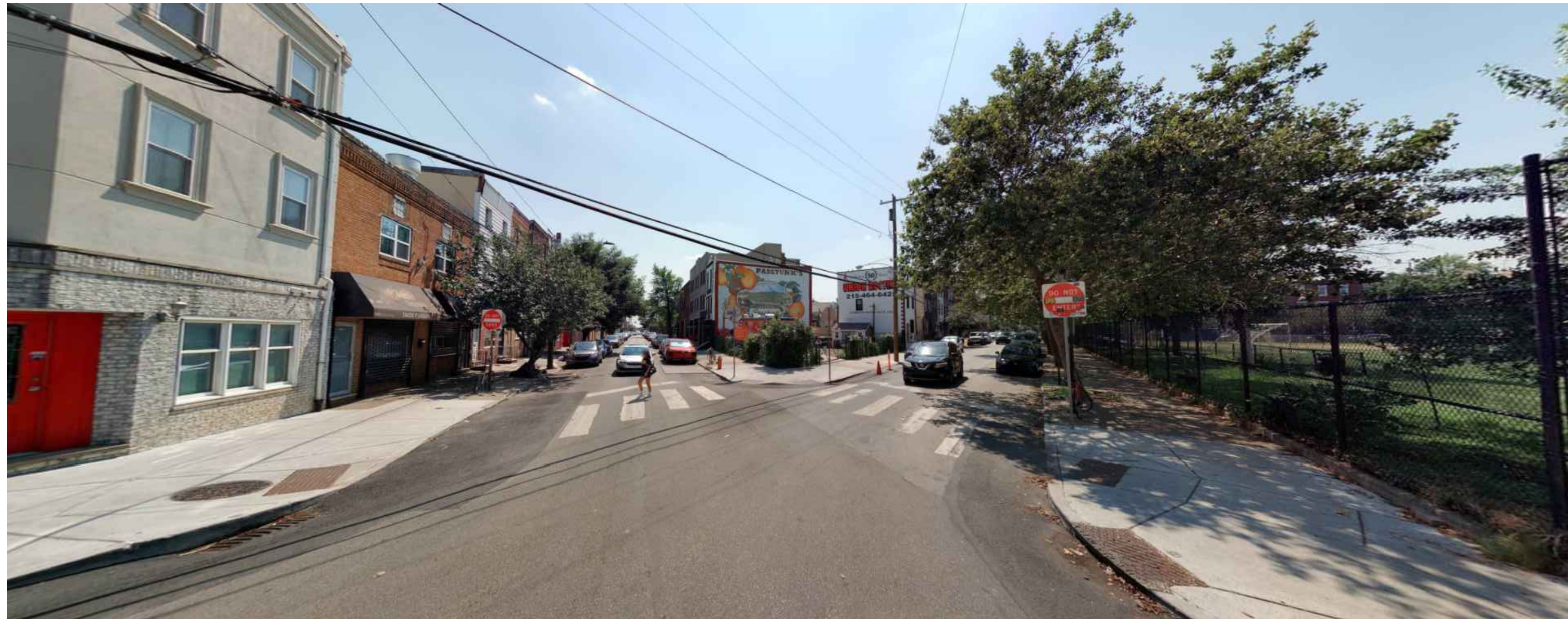
VIEW ACROSS THE STREET (WEST) ON E. PASSYUNK AVE
