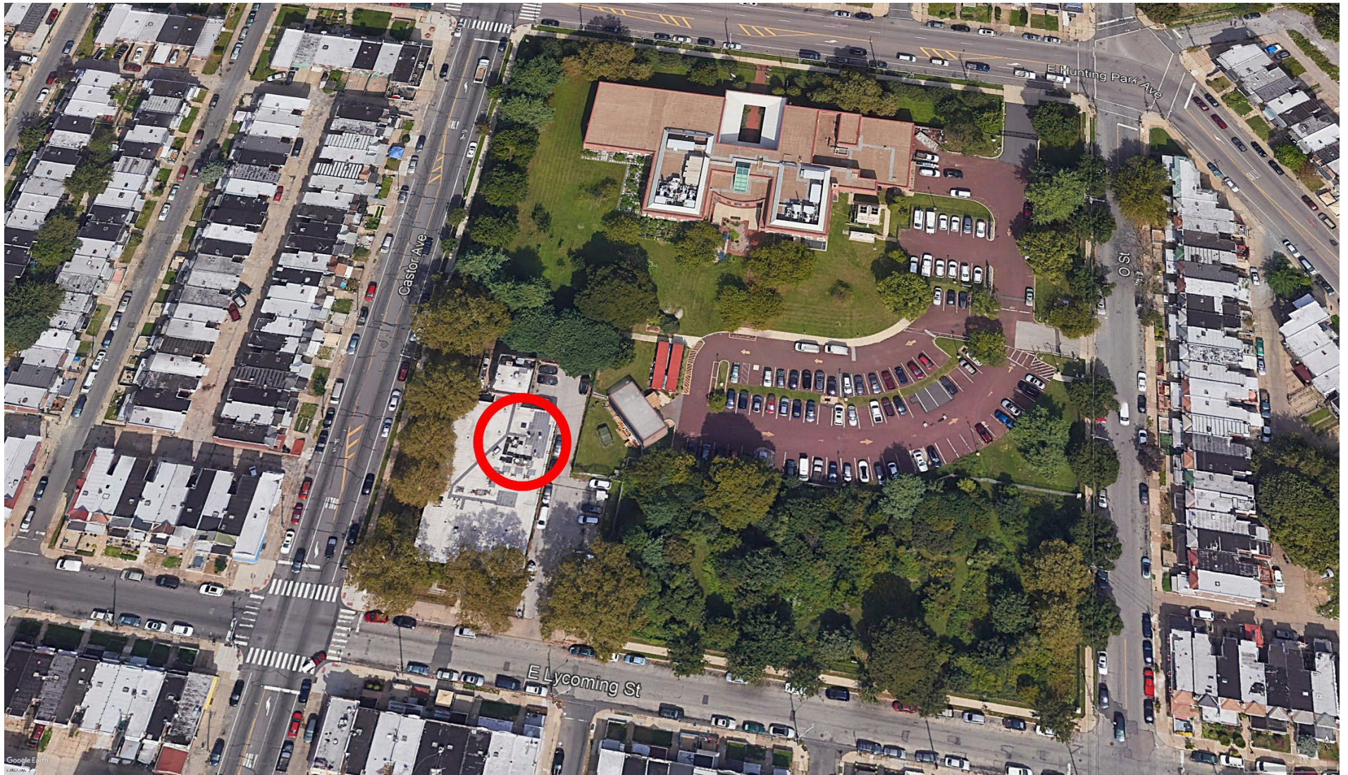
Figure 9 - LAB North Aerial View
