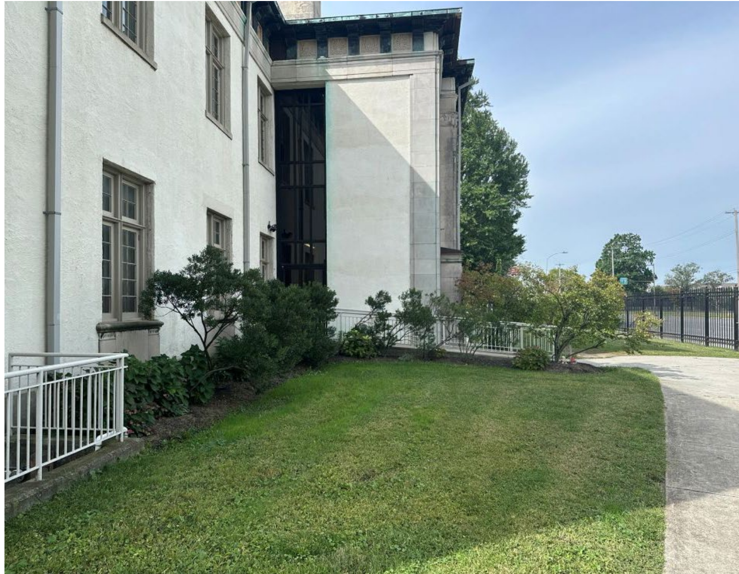
PATTISON AVE BUILDING ENTRY AND ACCESSIBLE RAMP
