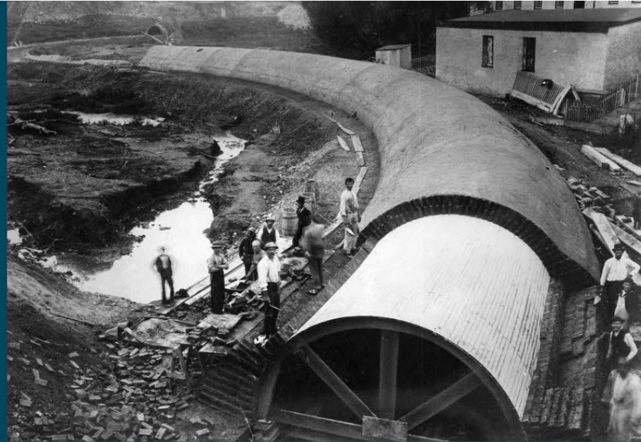
Mill Creek Culvert Construction and Funston St Collapse, courtesy Philadelphia Evening Bulletin, George D McDowell Collection, Special Collections Research Center, Temple University Libraries
