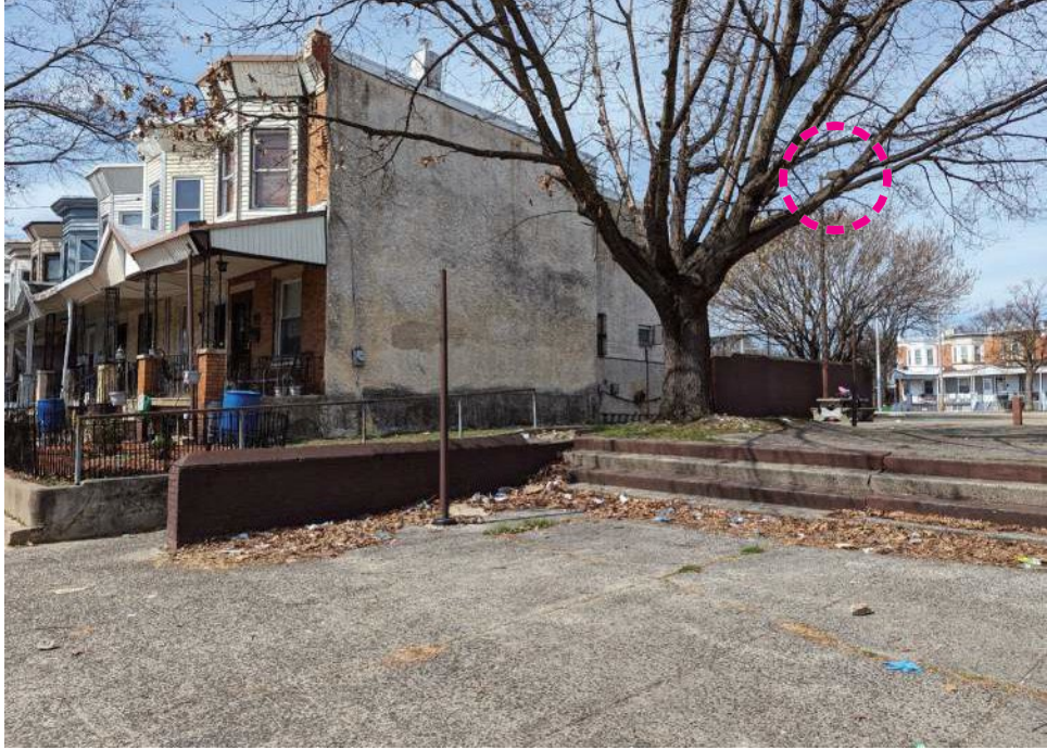
EXISTING POLE LIGHT FIXTURE TO BE REPLACED
