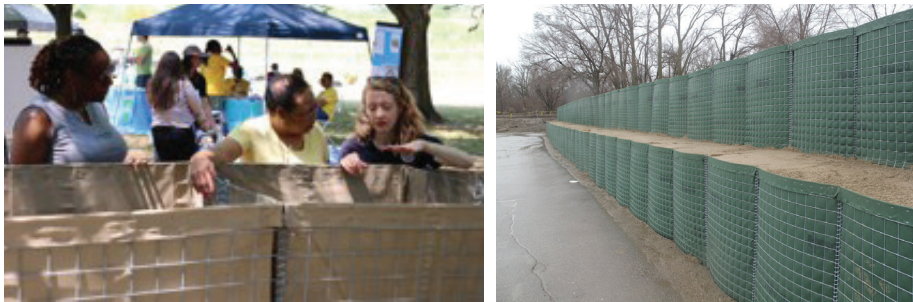
Demo barriers on display at Eastwick Community Day (above left) and an example of barriers stacked for flood protection (above right) Source: HESCO Bastion, Inc.
