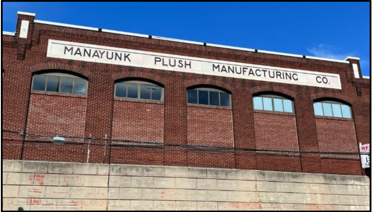
Figure 30. The permanent, attractively rendered signage of the Manayunk Plush Manufacturing Company is evocative of the location as well as the once prominent industry. Source: Oscar Beisert, 2025.
