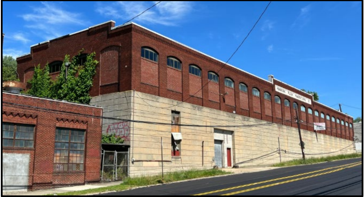
Figure 29. The northwest and southwest elevations of the Manufacturing Building. Source: Oscar Beisert, 2024.
