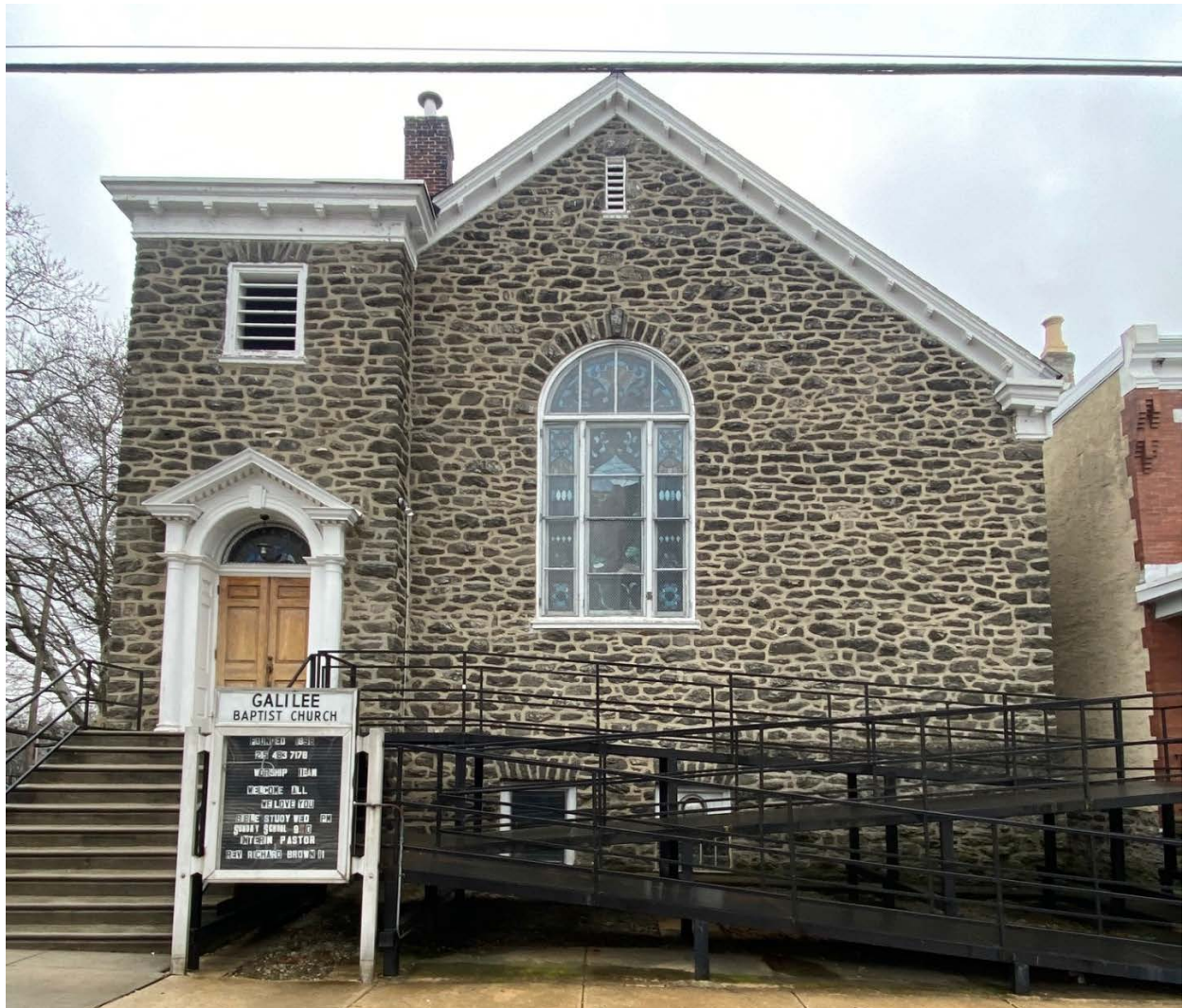
Figure 2. Galilee Baptist Church, 459 Roxborough Ave., Primary (north) façade, April 2026.
