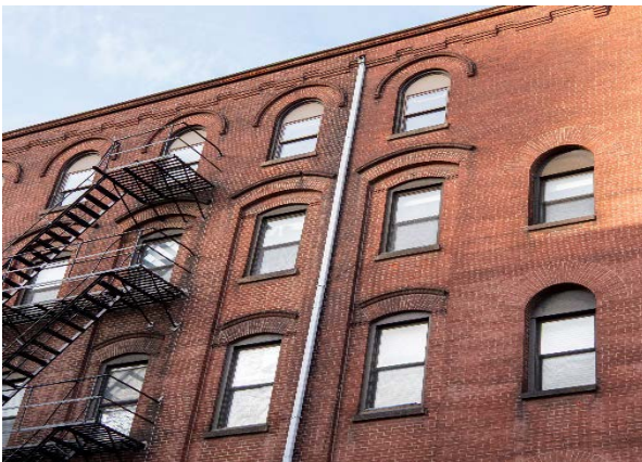
Figure 27. Segmental-arch lintels
