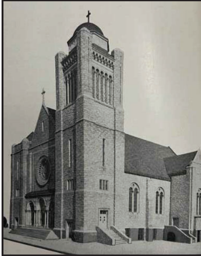
Figure 40. The primary (northwest) and side (southwest) elevations in ca. 1945. Source: CHCR.
