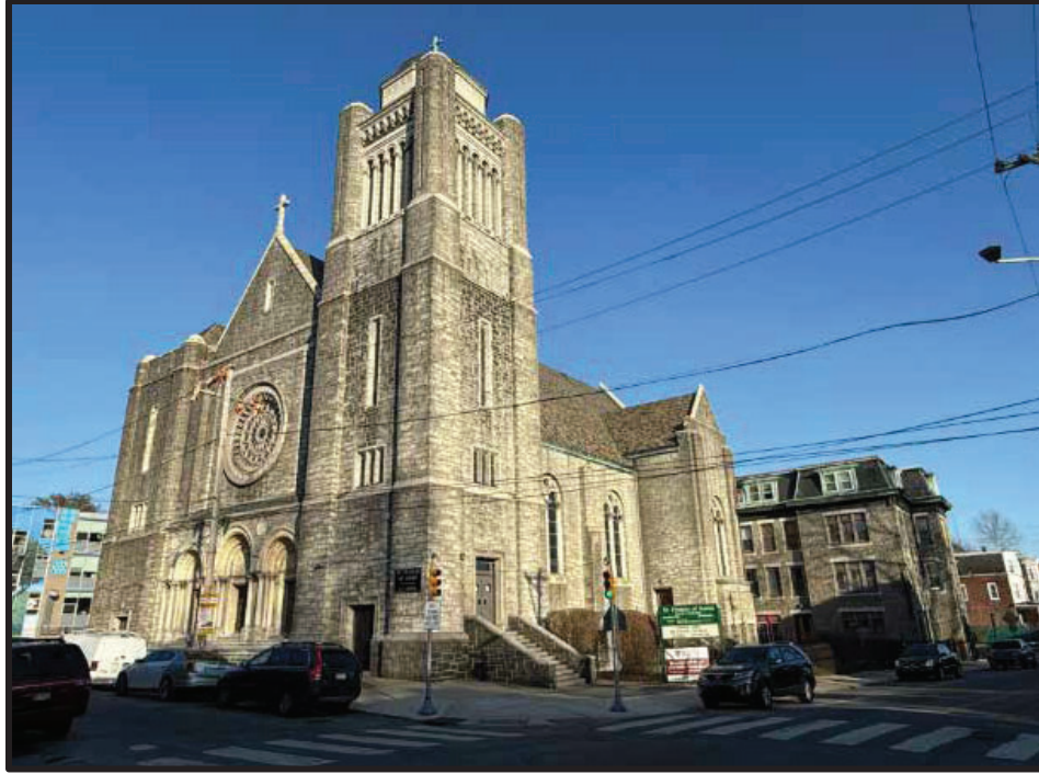
Figure 2. The primary (northwest) and side (southwest) elevations. Source: Oscar Beisert, 2026.
