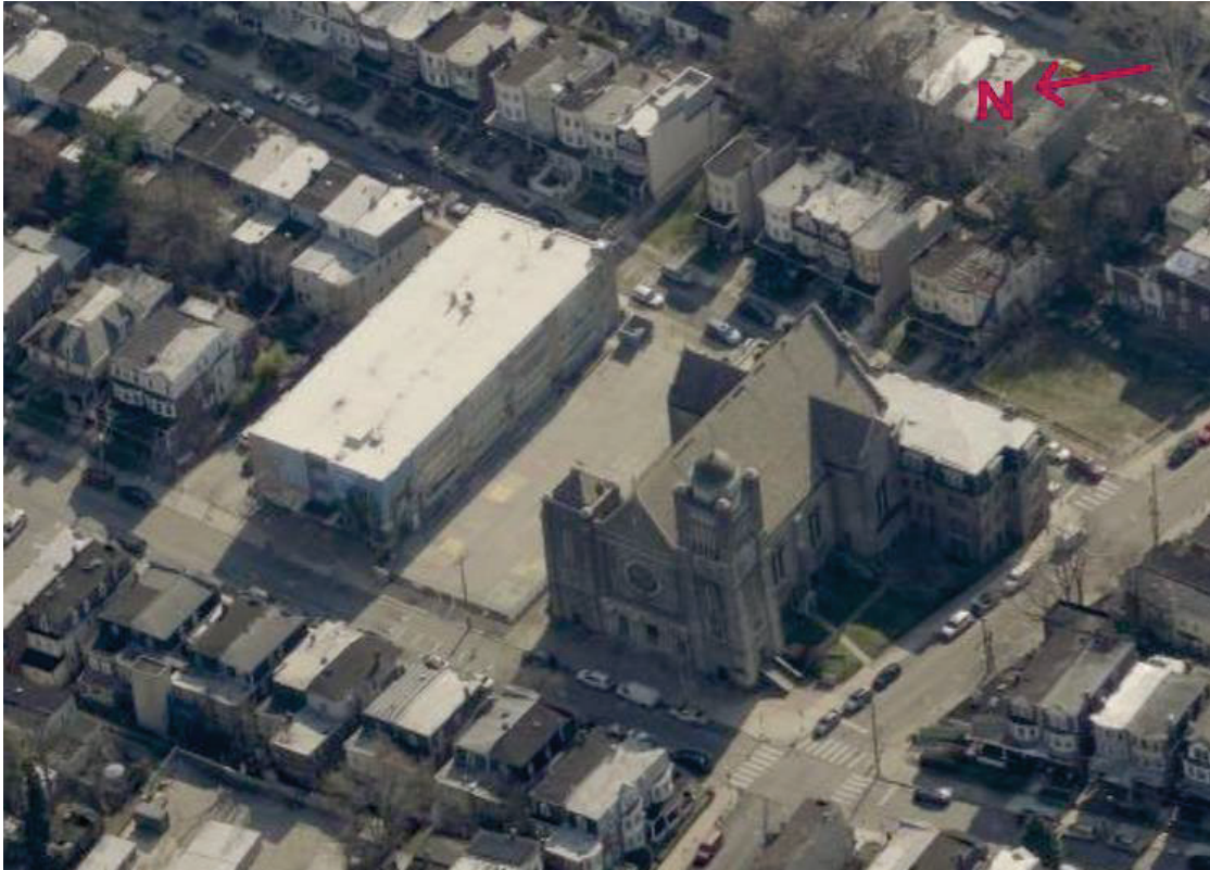
Image 2: Aerial view from the west of St. Francis of Assisi Roman Catholic Church complex at 48-60 W Logan St., showing the church and rectory (right) and school (left). From Cyclomedia.
