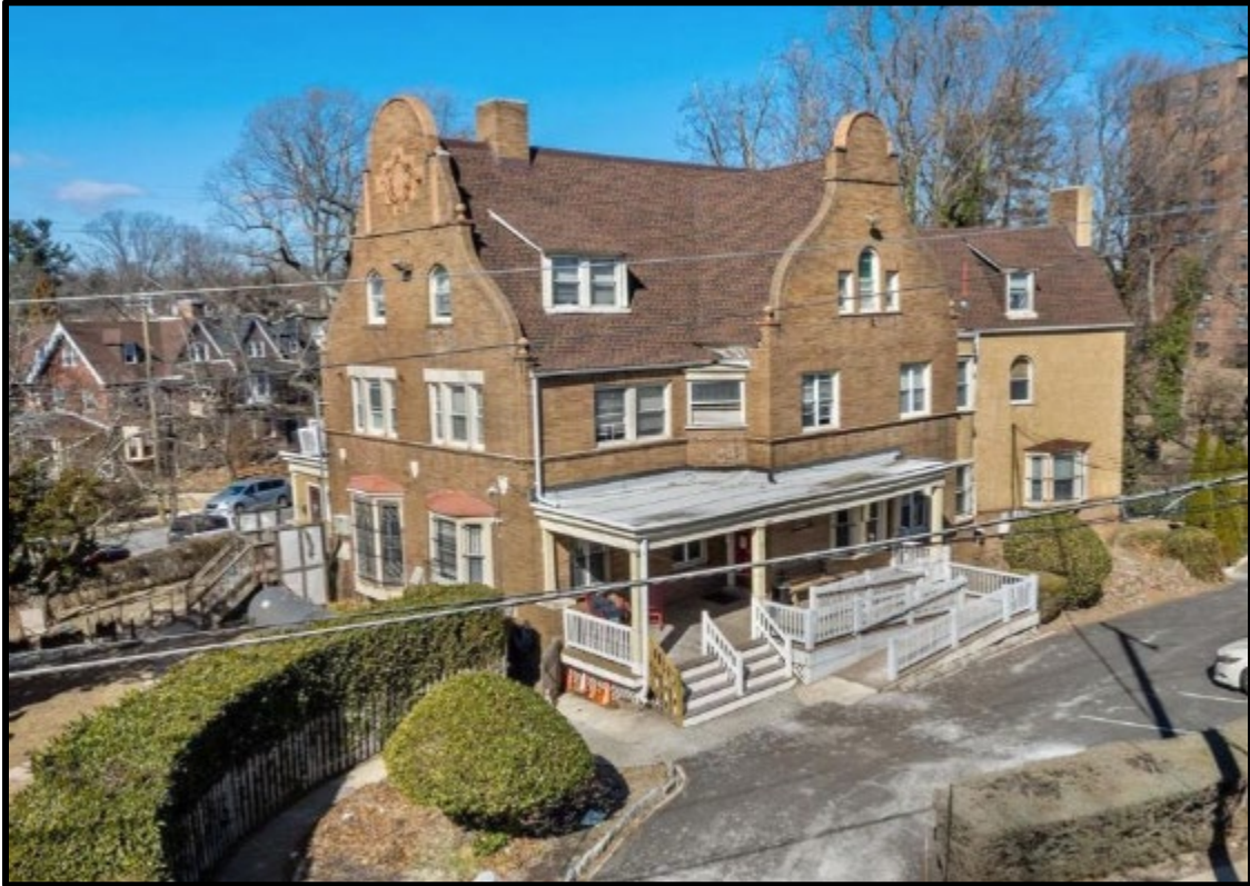
Figure 1. The south and east elevations. Source: Google, 2025.
