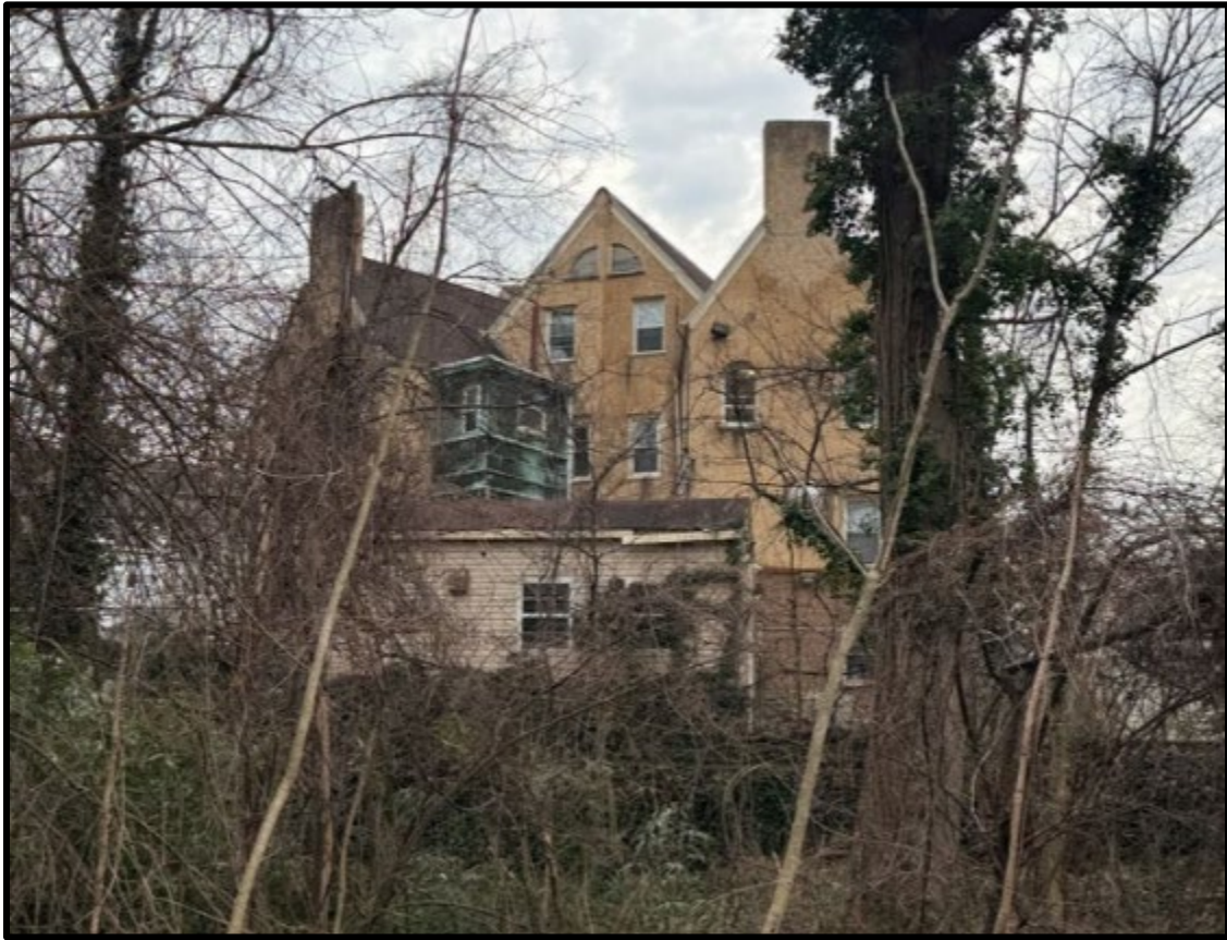
Figure 9. The rear (north) elevation. Source: Keeping Society of Philadelphia, 2026.
