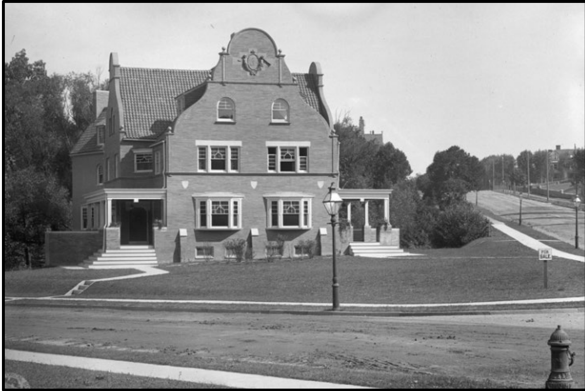
Figure 13. The primary (south) elevation in ca.1895-1900. Source: Radnor Historical Society.
