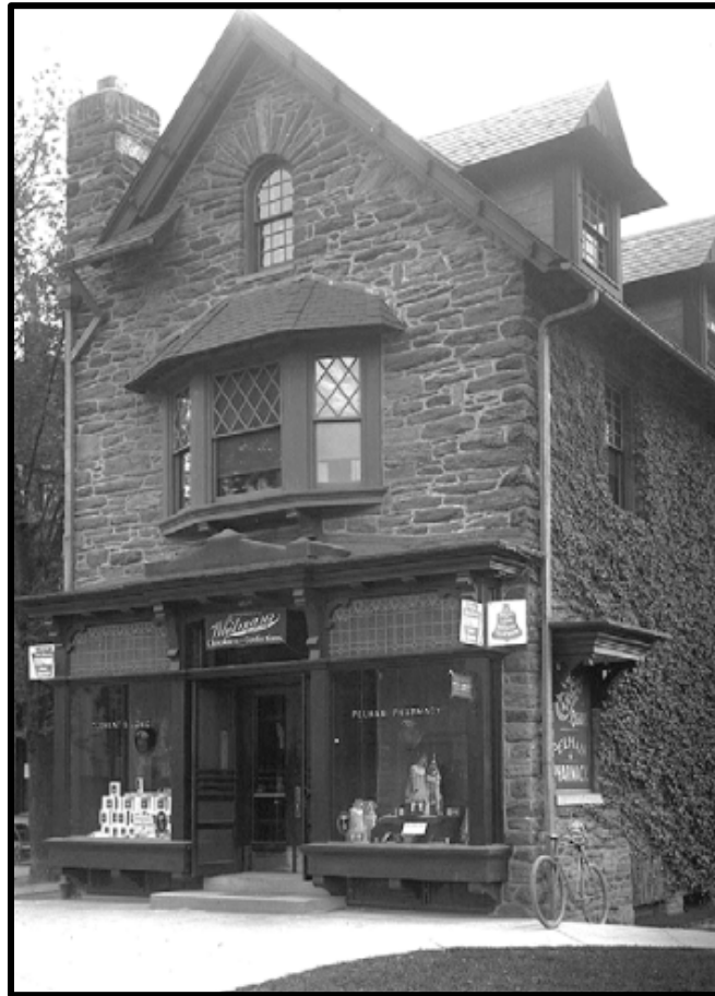
Figure 26. The Pelham Pharmacy, 6626 Germantown Avenue, Pelham, West Mount Airy, designed by David Knickerbocker Boyd in 1904. Source: Free Library of Philadelphia.
