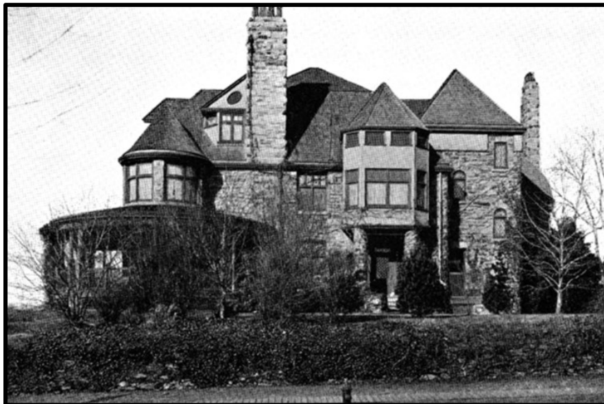
Figure 15. “Uwchllan,” the Cornelius N. Weygandt House (Demolished), West Upsal Street. Source: Germantown Historical Society.
