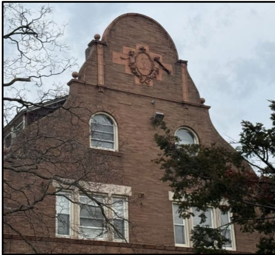
Figure 4. The upper portion of the Flemish gable in the primary (south) elevation. Source: Keeping Society of Philadelphia, 2026.
