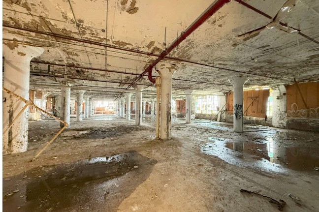
Photo 10: Interior: third floor, looking south.
