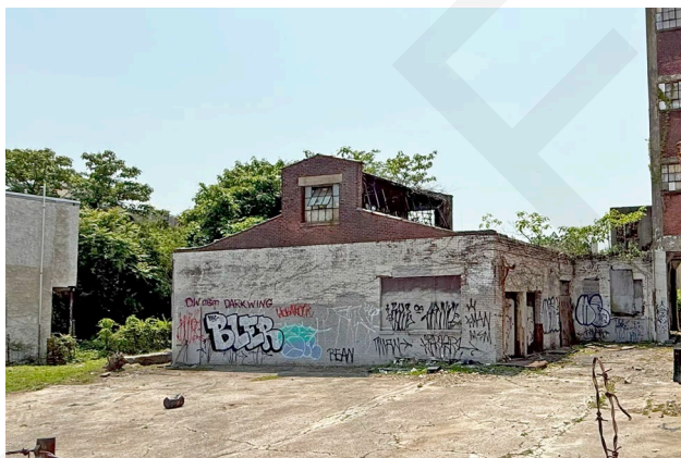
Photo 13: Boiler House, south and west elevations, looking southeast.
