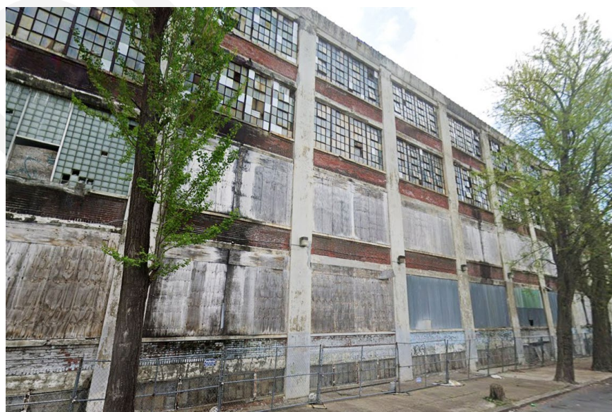
Photo 2: West elevation, looking southeast.
