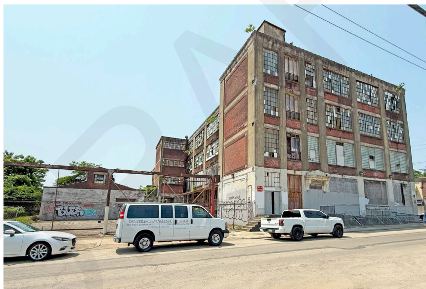
Photo 5: East and north elevations, looking southwest.
