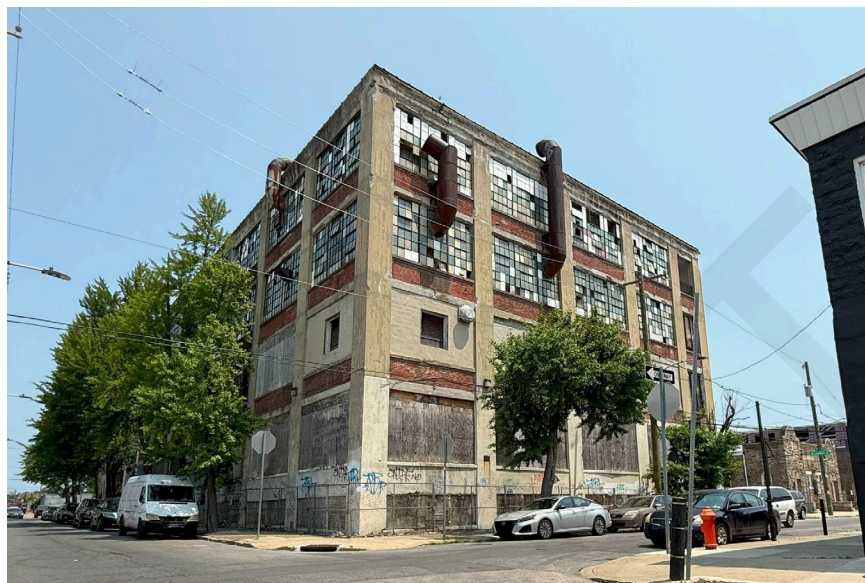
Photo 3: West and south elevations, looking northeast.
