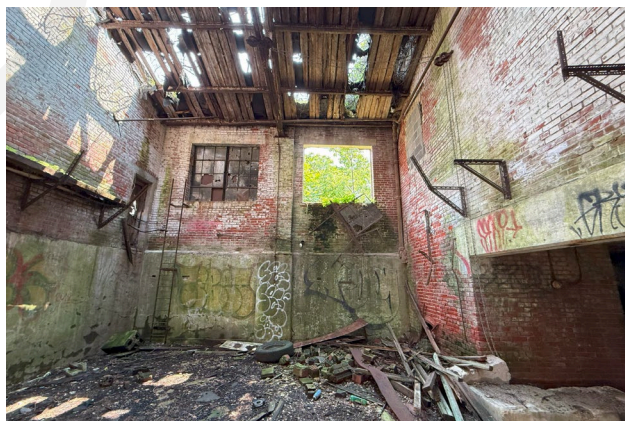
Photo 14: Boiler house, interior of northern section, looking south.
