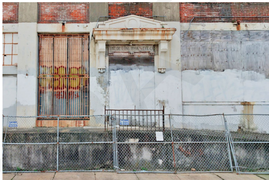
Photo 6: North elevation, close-up view of historic main entrance, looking south.
