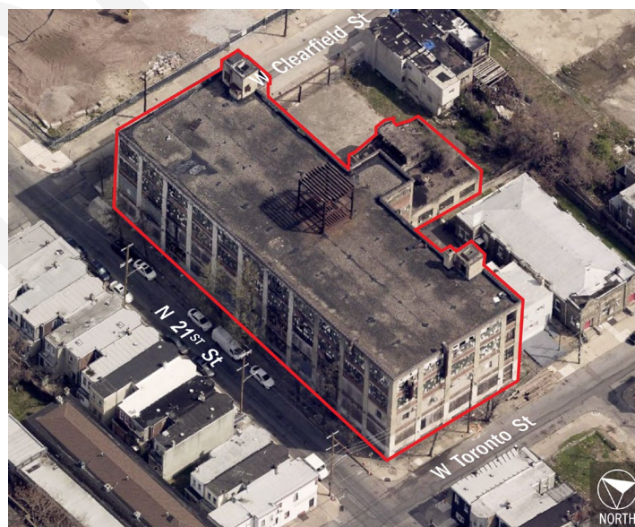
Figure 2: Recent aerial view, looking northwest (Imagery from Pictometry).
