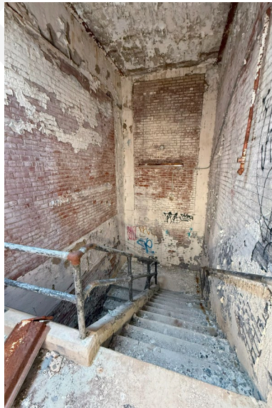
Photo 12: Interior: Egress stair in south tower, fourth floor, looking north.
