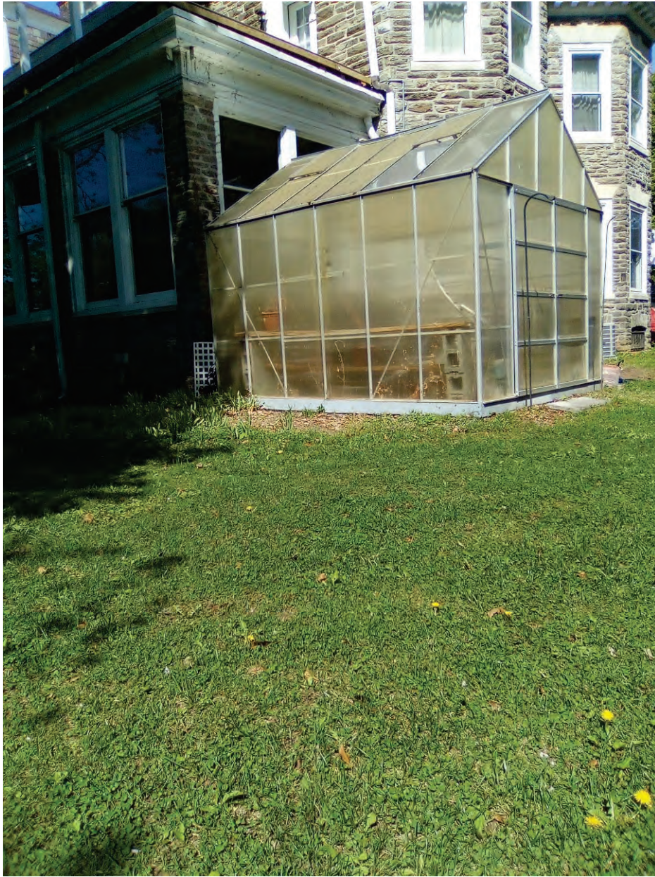
Preferred location of proposed exterior staircase (behind greenhouse structure).
