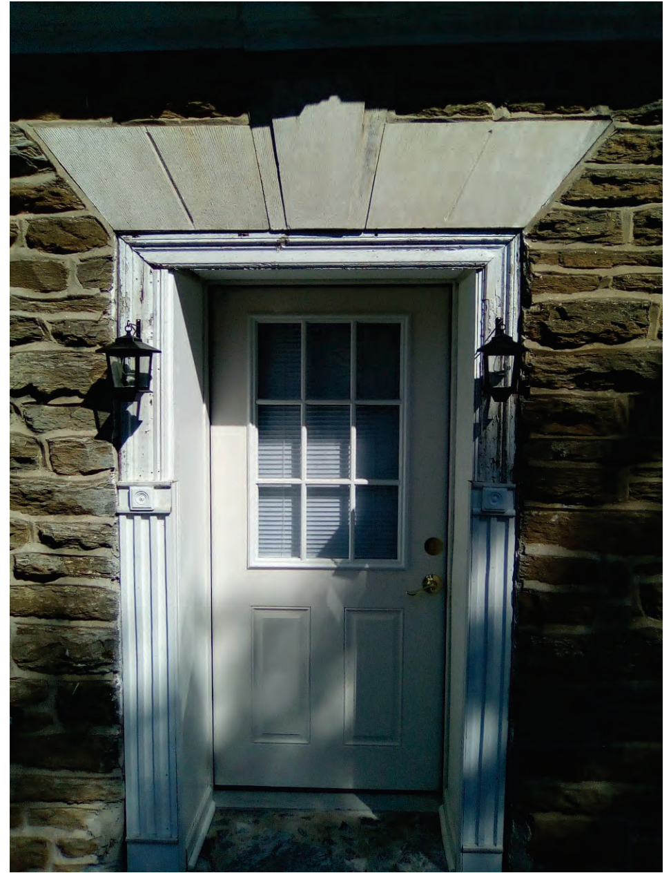
Photographs of doors installed in altered window openings on second story.
