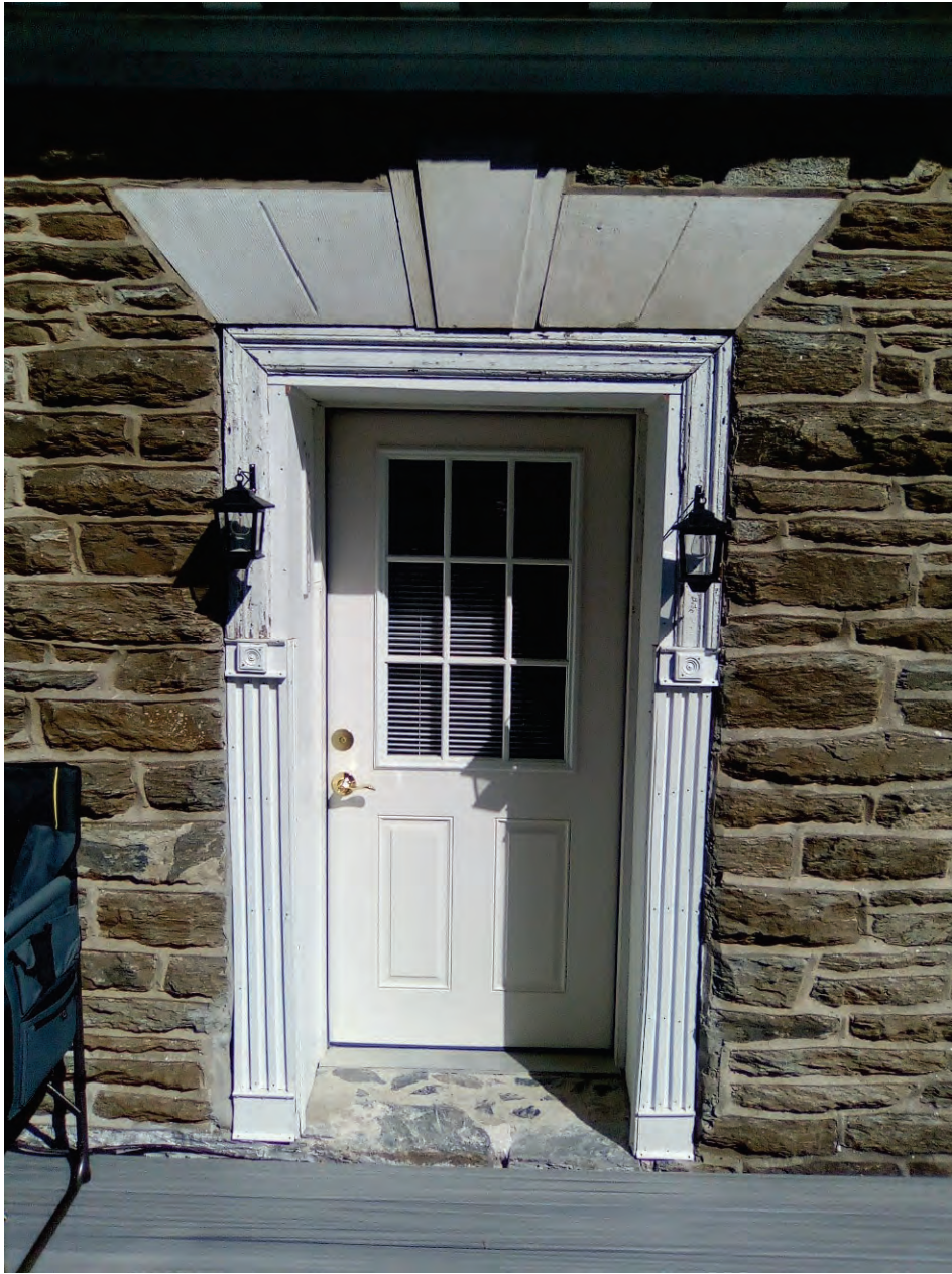
Photographs of doors installed in altered window openings on second story.
