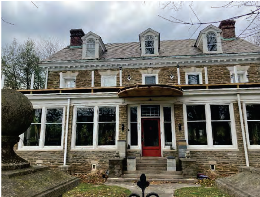
Image 4: 6363 Overbrook Ave, showing extent of work completed, on 3/30/2026.
