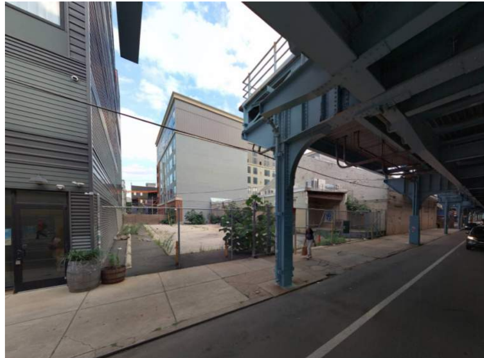
5 SOUTHEAST VIEW FROM N. FRONT ST.
