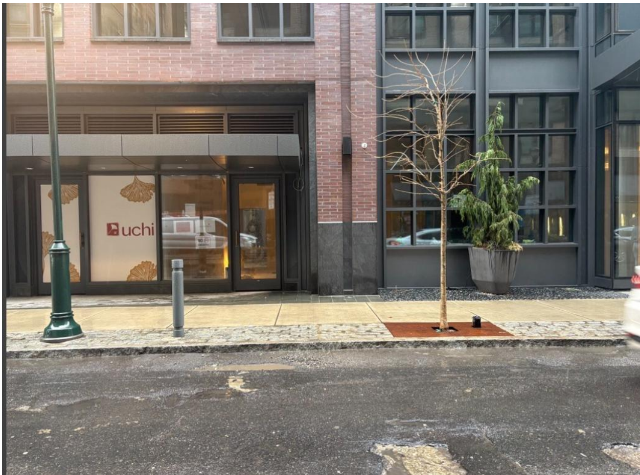
PHOTO #1A – Façade
