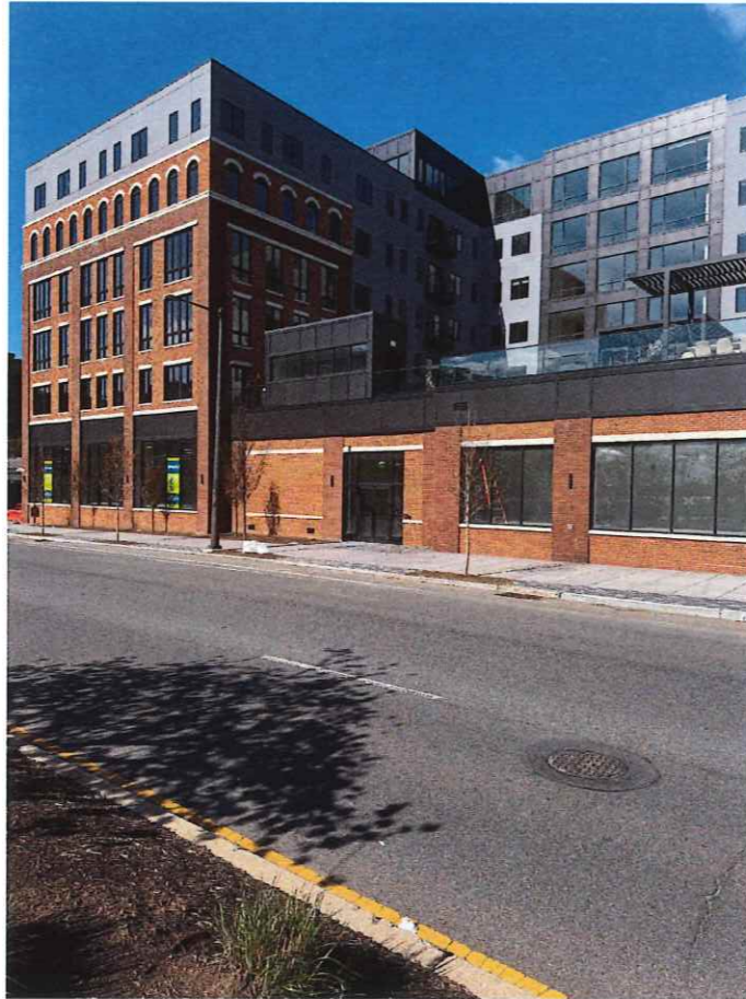
Signs EO1.7 & EO1.8 Delaware Avenue – building to left
