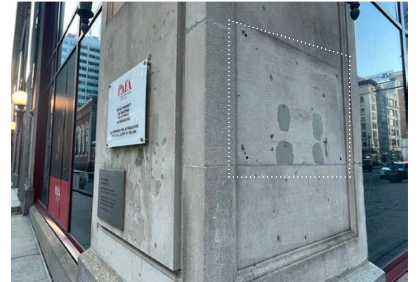
Covers visible masonry patches.
