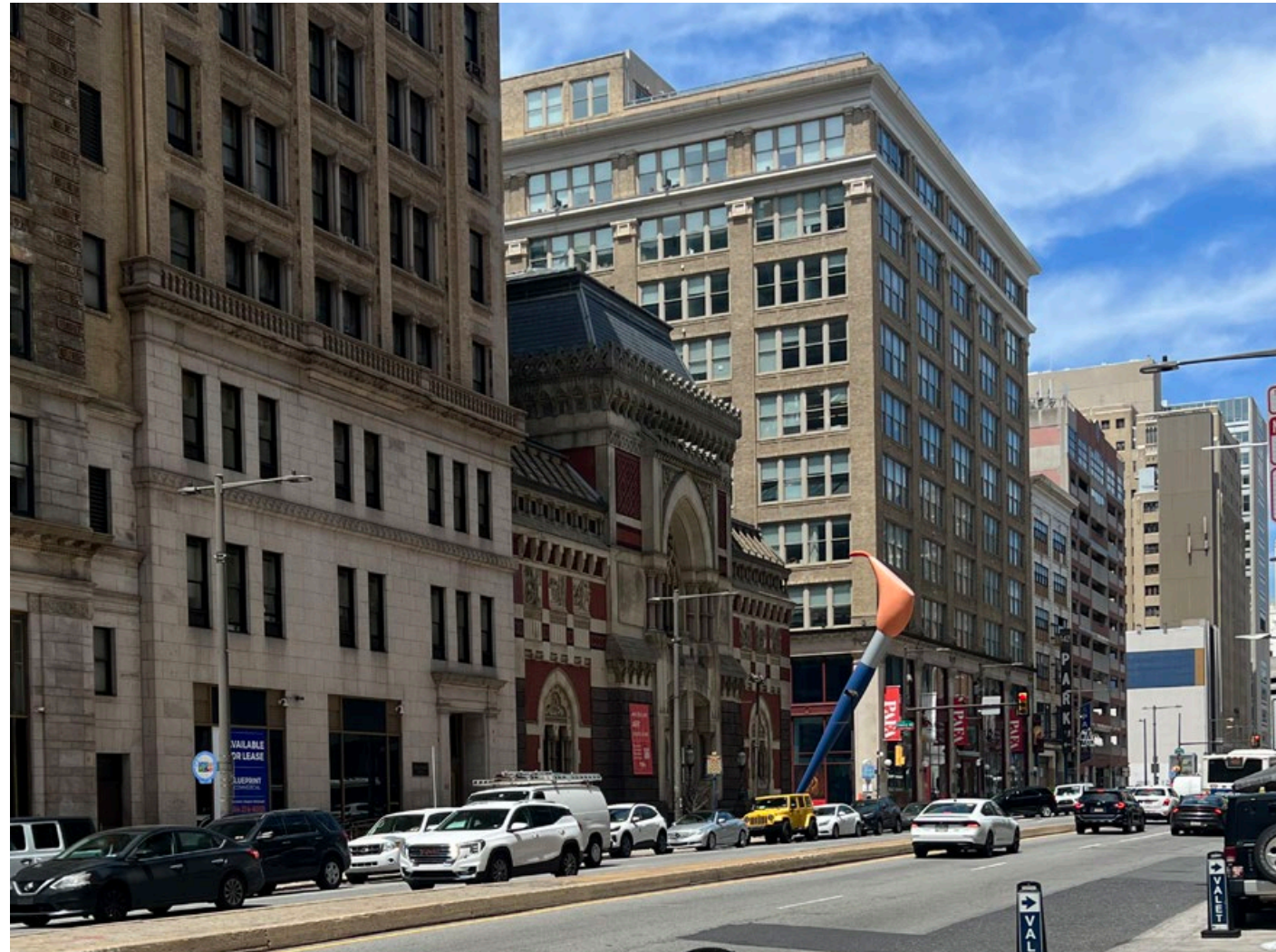
On Broad Street Facing North-West
