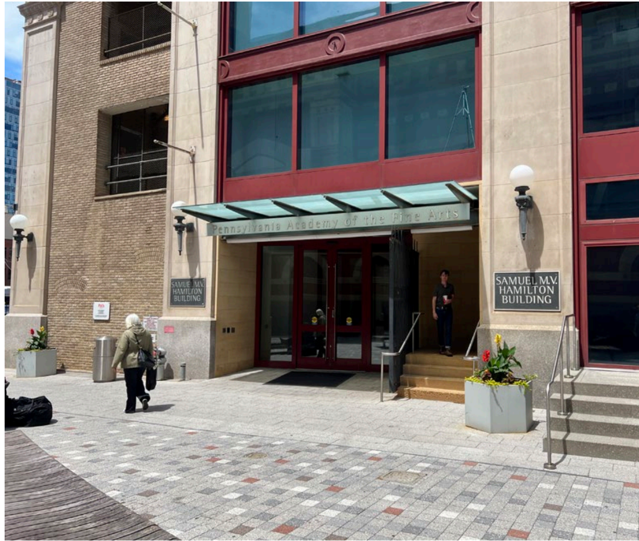
In Lenfest Plaza Facing North
