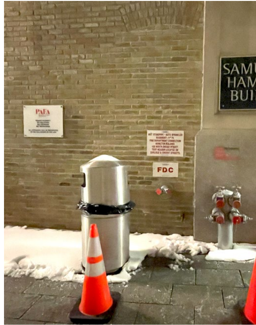
In Lenfest Plaza Facing North
