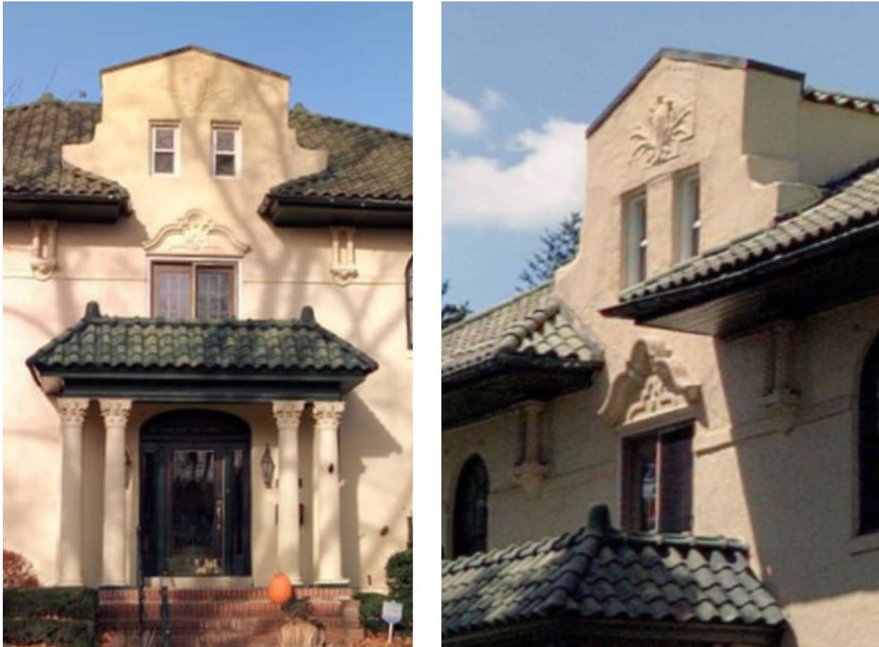
Figure 9. The front dormer extends up from the front façade and serves as an espadaña or curved parapet. Decorative Spanish Baroque reliefs ornament the façade above the French doors and at the espadaña.
