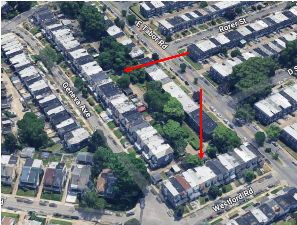
Figure 23. Carl Metz constructed 58 two-story rowhouses on the east side of the 5300-block of Westford Street and the south side of the 500-block of Geneva Avenue in the mid 1920s.
