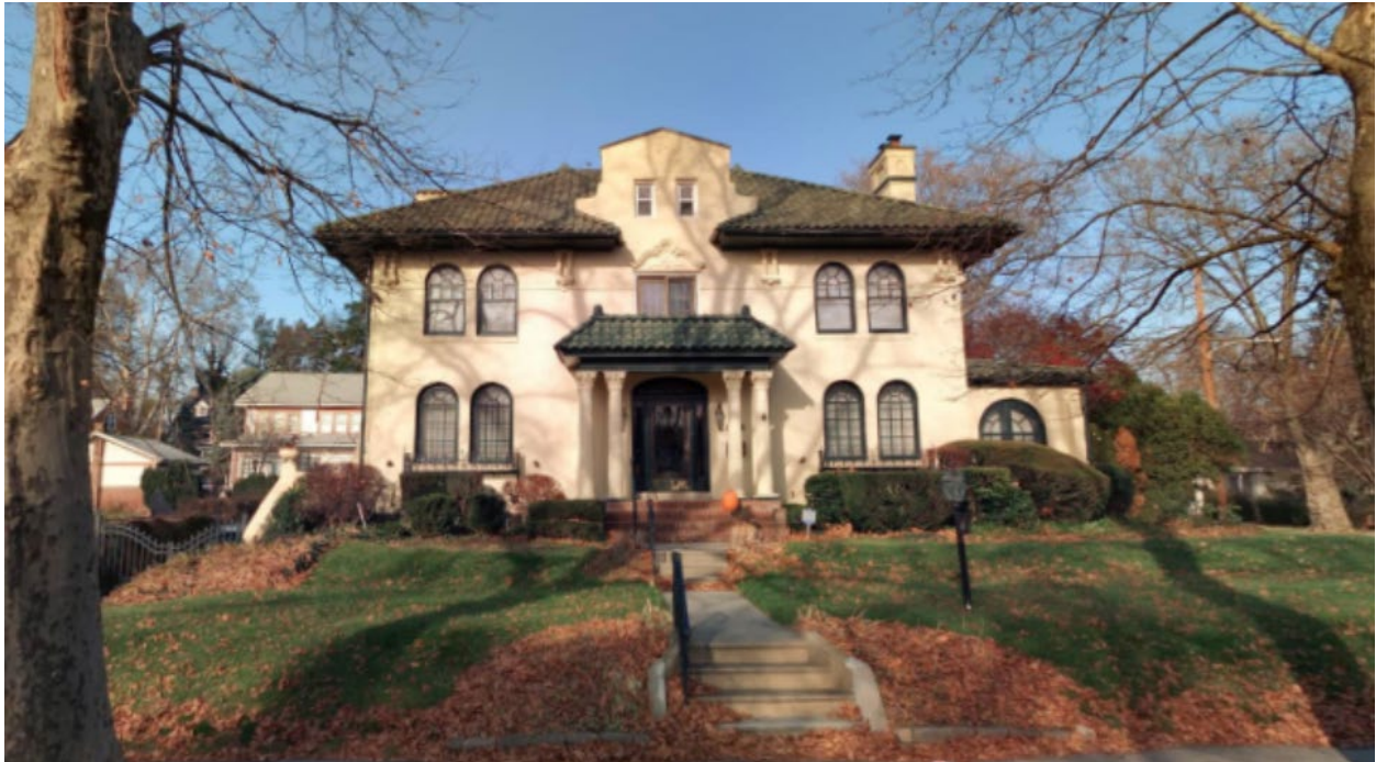
Figure 4. View of the house at 601 W. Godfrey Avenue looking north, December 4, 2022. Source: Cyclomedia.
