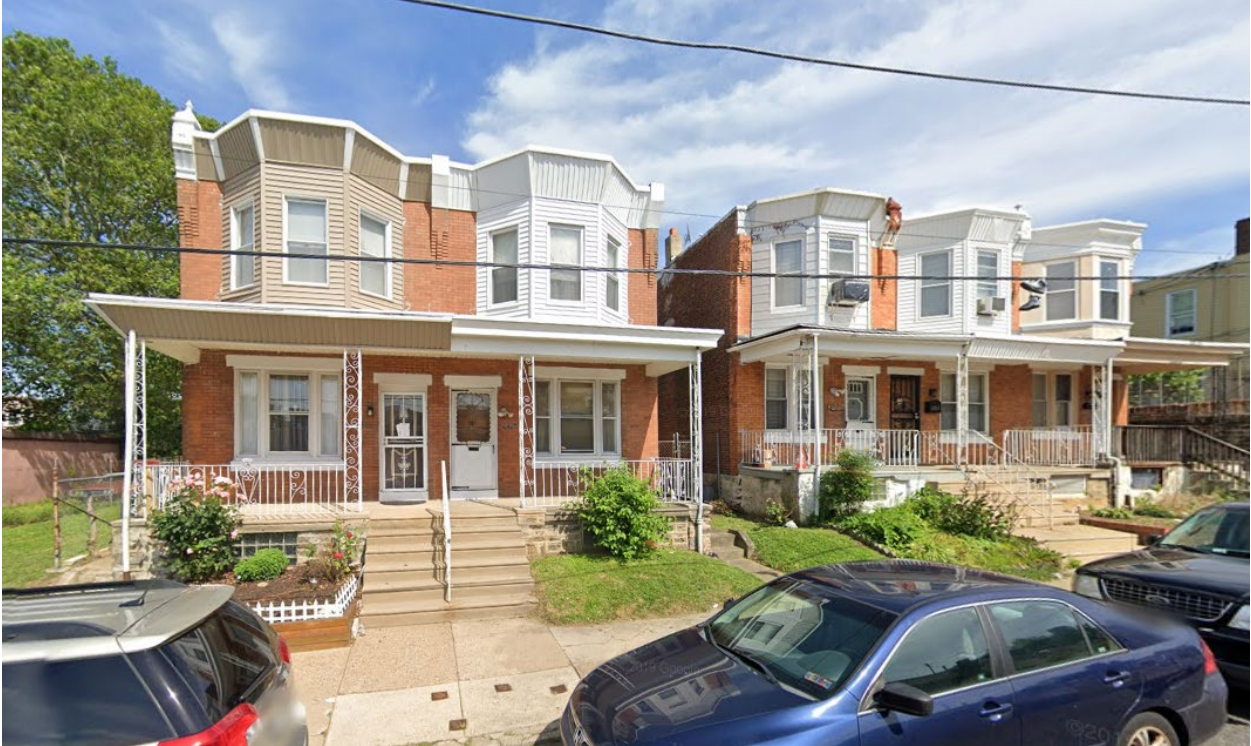
Figure 15. Carl Metz developed the houses at 4901 to 4909 N. Lawrence Street in 1914 and 1916.
