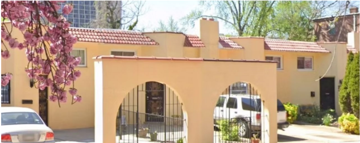
Figure 115. Spanish Village, 2000-2014 Green Street, Spring Garden, Mariano E. Martinez, architect, 1972.
