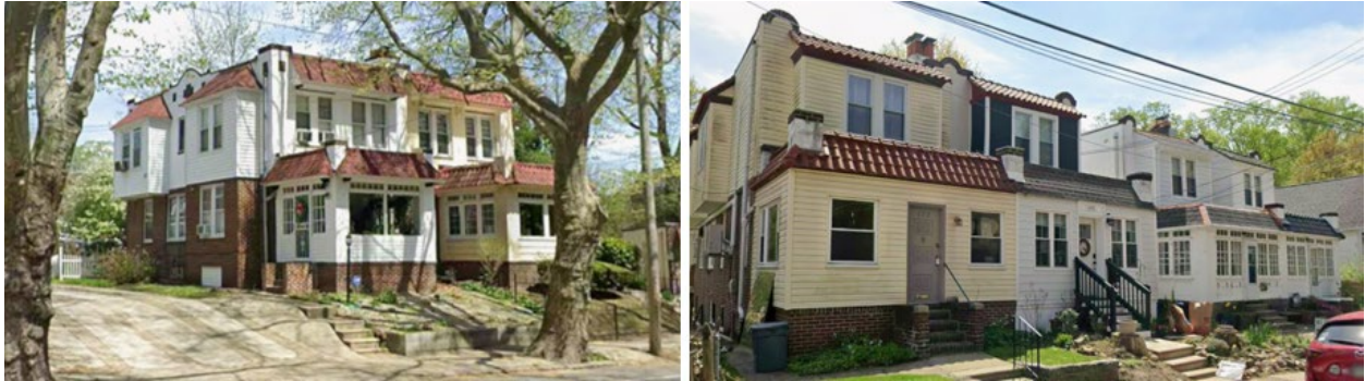
Figure 81. Spanish-type twins 881 to 887 W. Walnut Lane and 693 to 699 W. Johnson Street, Fred N. Greisler, architect, 1925.
