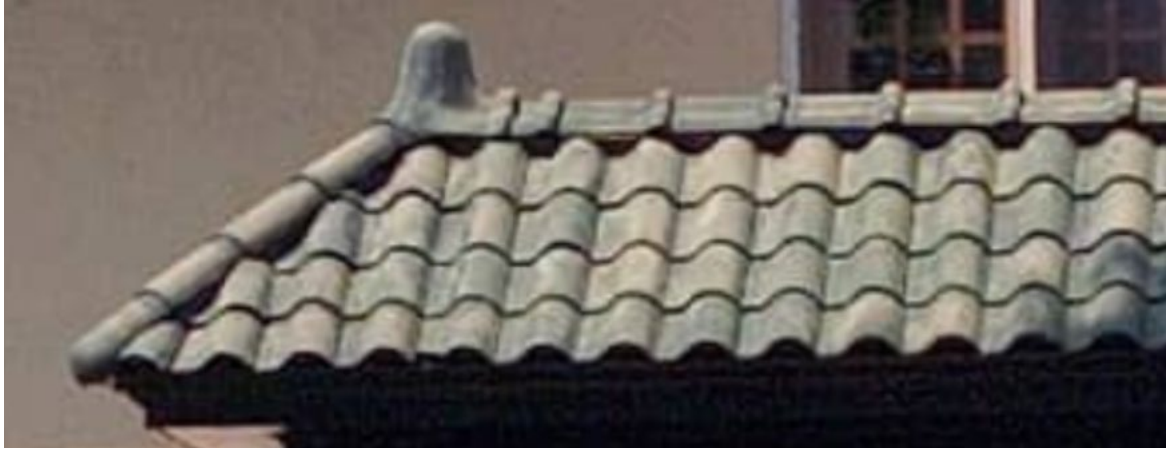
Figure 10. Green Spanish barrel tile on the front porch at 601 W. Godfrey Avenue.
