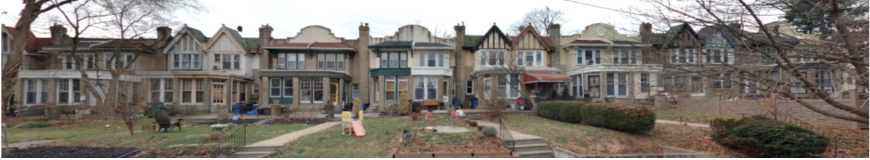
Figure 31. A section of the English and Spanish row at 5046 to 5084 McKean Avenue, Germantown, constructed by John J. Bateman & Sons, 1926.
