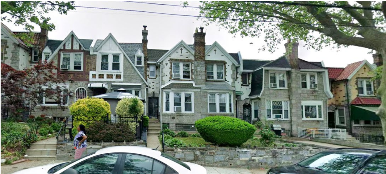
Figure 46. “English” houses with front facades clad with North Carolina granite on the 5200-block of C Street in the Olney neighborhood, constructed by Carl Metz Jr. in 1930.
