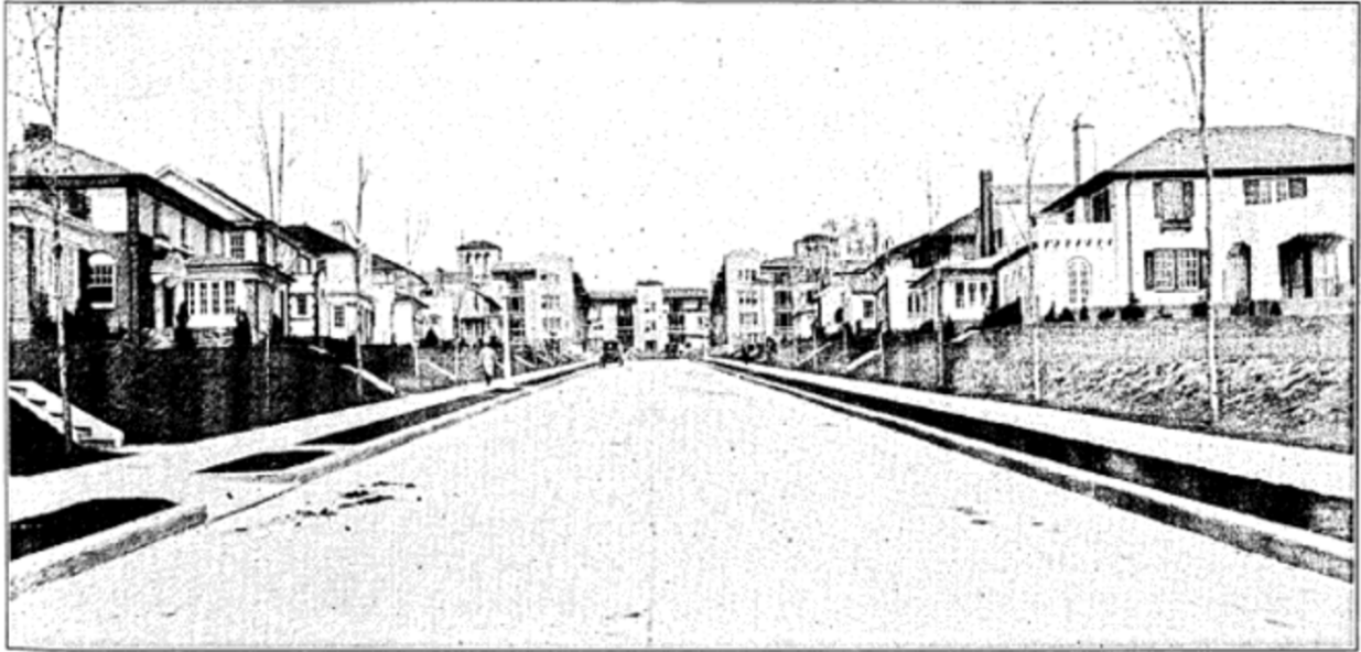
Figure 99. A view up Elkins Avenue to the Elkins Court apartment building, from "Elkins Park, An All-Concrete Development," Concrete , v. 31, n. 4, October 1927, p. 43.
