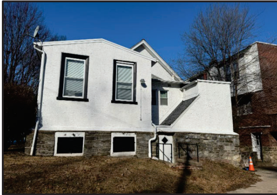
Figure 5. The rear (southeast) elevation, including the three additions. Source: Oscar Beisert, 2025.
