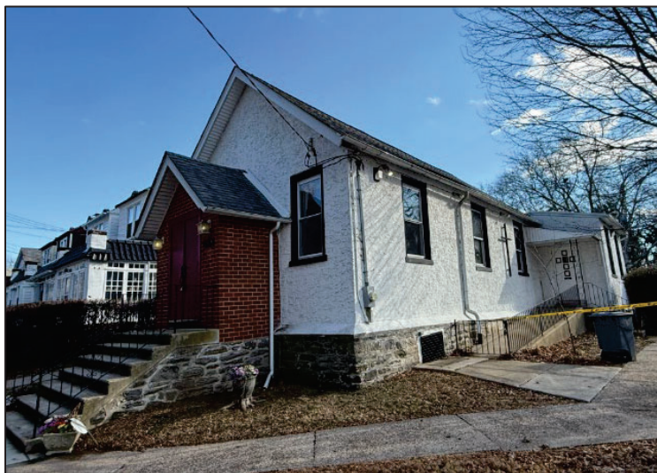
Figure 4. The primary (northwest) and side (southwest) elevations. Source: Oscar Beisert, 2025.
