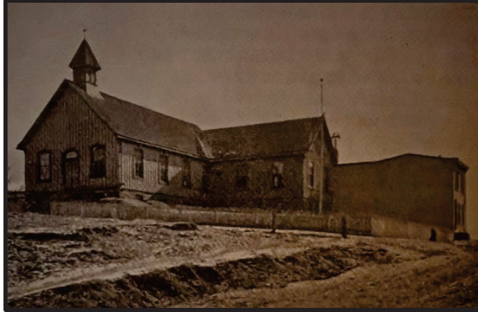
Figure 23. The frame chapel of Emmanuel Methodist Episcopal Church in 1894. Source: Oscar Beisert . Philadelphia Register of Historic Places Nomination: Gates Street Historic District. ( Philadelphia: Ridge Park Civic Association, 2022 ).
