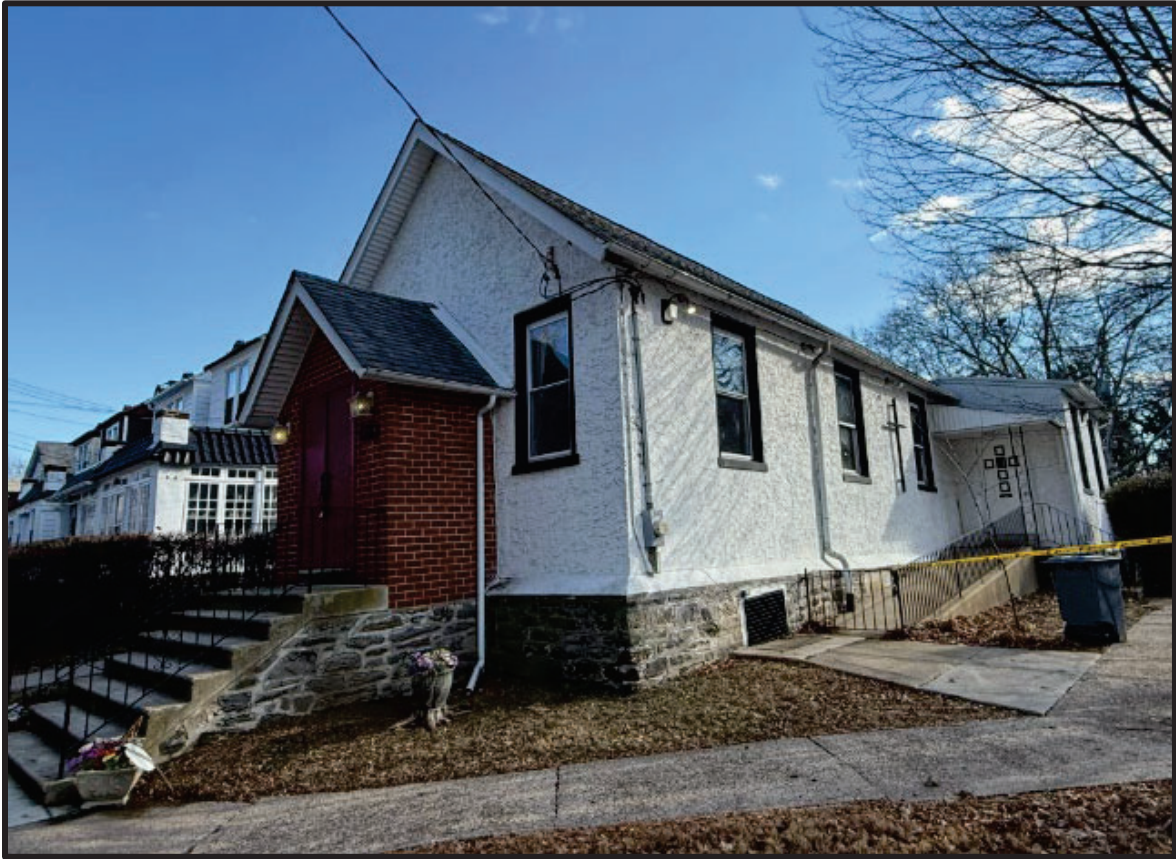
Figure 1. The primary (northwest) and side (southwest) elevations. Source: Oscar Beisert, 2025.
