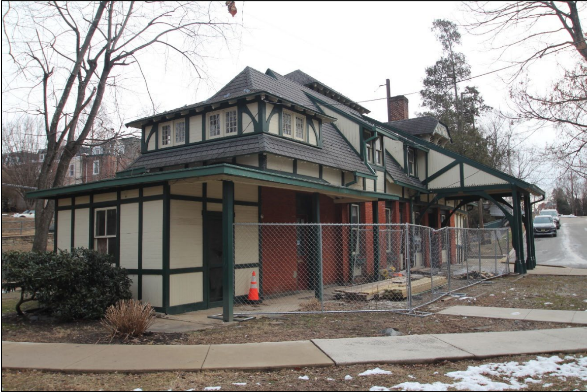
Photo 4: 119 East Gowen Ave, southwest elevation, looking east. (Robert Powers, 2025)
