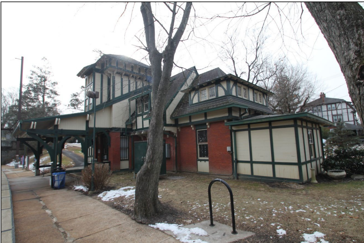
Photo 3: 119 East Gowen Ave, southwest elevation, looking north. (Robert Powers, 2025)
