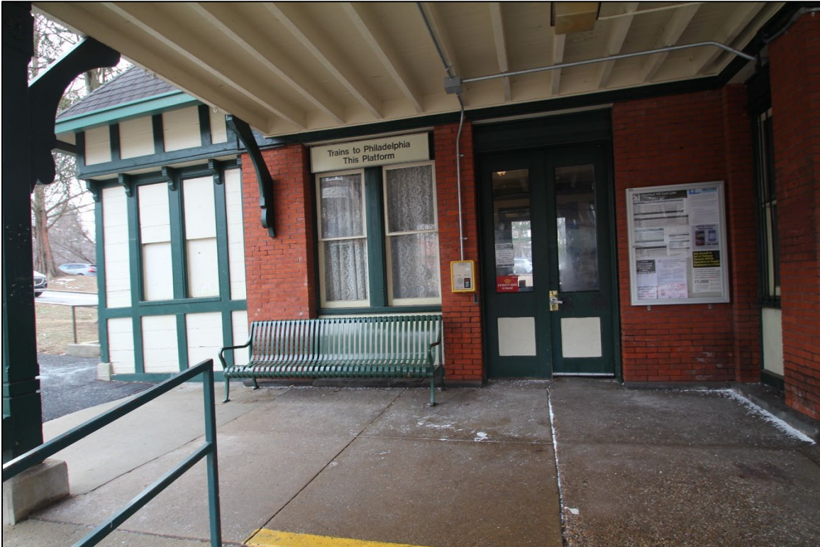
Photo 2: 119 East Gowen Street, northeast elevation, showing the door to the waiting room, looking southwest from the platform. (Robert Powers, 2025)
