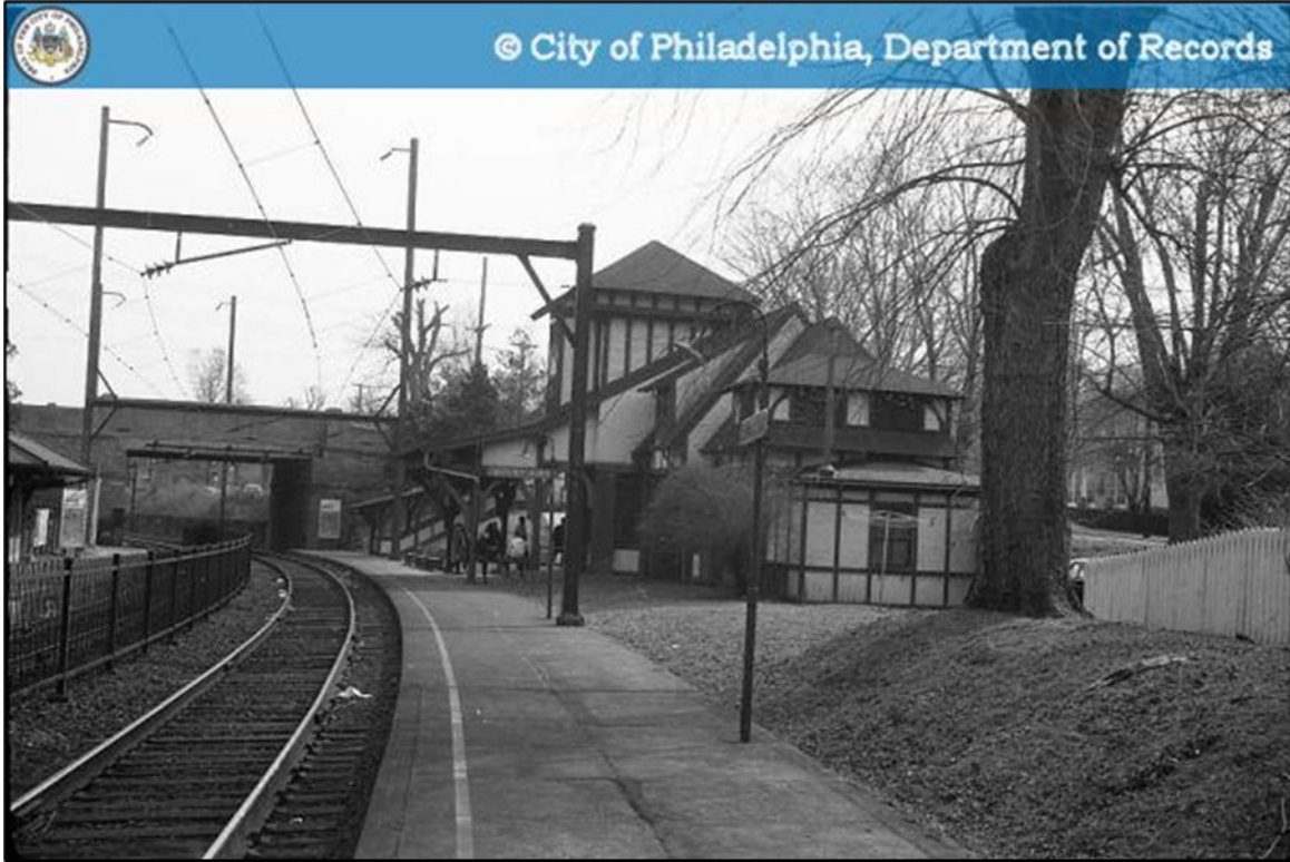
Figure 3: 119 East Gowen Street seen from the northwest, 1963. The roof over the stairs to the platform has been modified, the stairs by the street are still present. (PhillyHistory.org)
