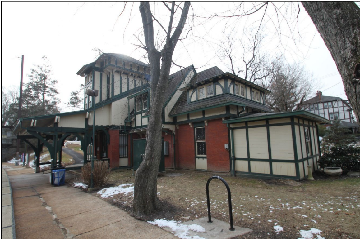
Photo 1: 119 East Gowen Street looking southeast from the platform. (Robert Powers, 2025)
