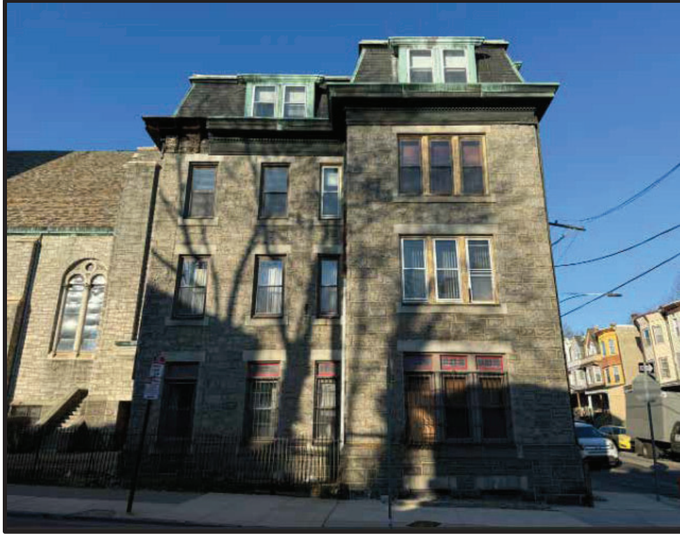
Figure 12. The southeast elevation of the Rectory. Source: Oscar Beisert, 2026.
