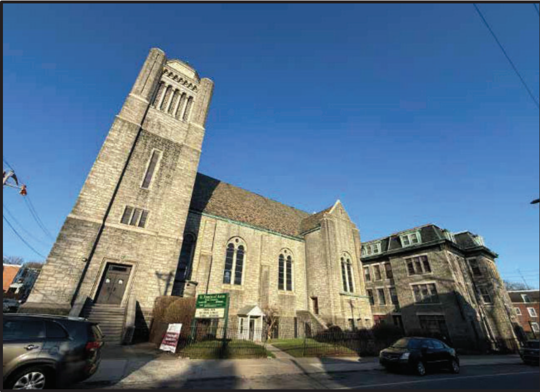
Figure 9. Top: The side (southeast) elevation. Figure 10. Bottom: The side (southeast) elevation. Source: Oscar Beisert, 2026.
