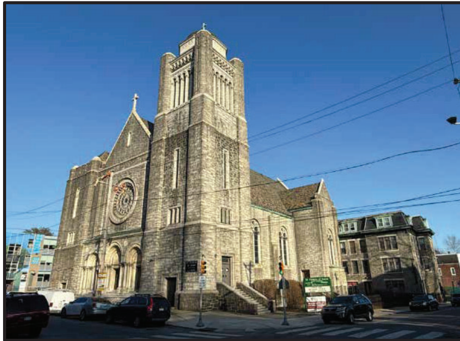
Figure 1. The primary (northwest) and side (southwest) elevations. Source: Oscar Beisert, 2026.
