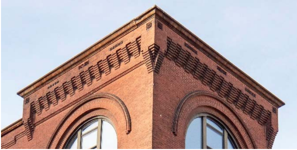
Figure 25. Brick-corbelled cornices
