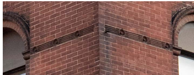
Figures 28 and 29. Terra cotta belt course, ornamental bands, and running bond brickwork
