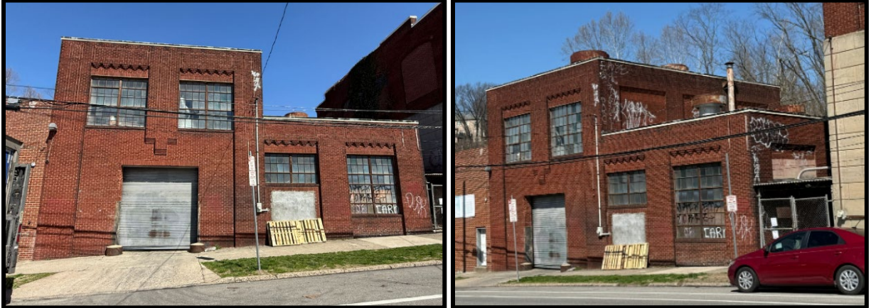
Figure 9. Left: The southwest elevation of the Power Plant. Figure 10. Right: The southwest and southeast elevations of the Power Plant. Source: Oscar Beisert, 2026.
