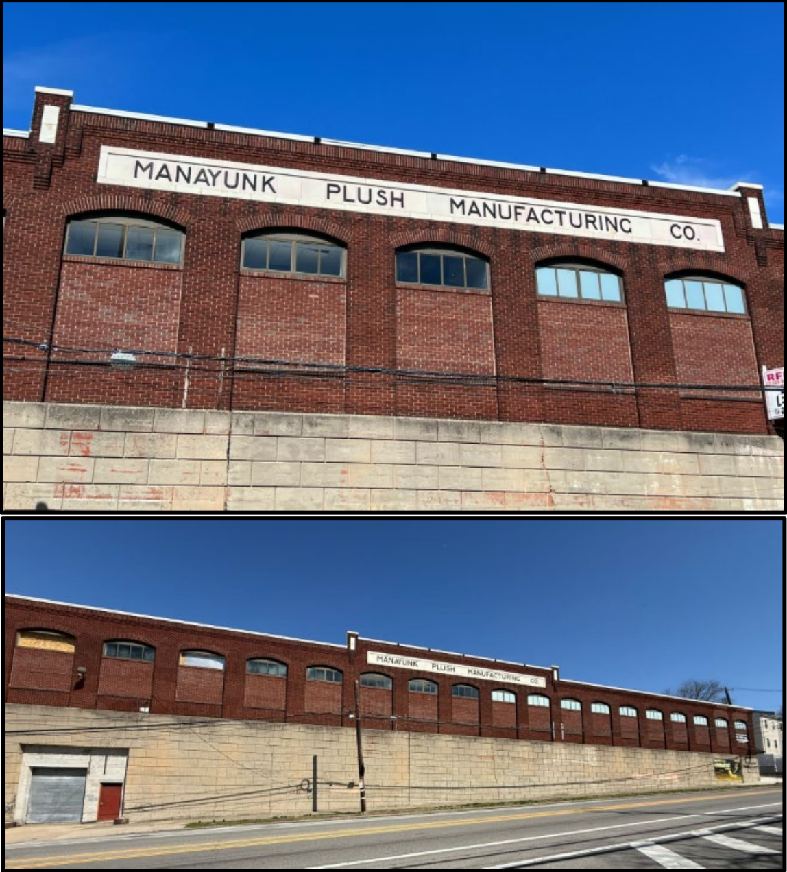
Figure 5. Top: The central bays of the southwest elevation, showing distinctive signage. Figure 6. Bottom: The southwest elevation along Umbria Street. Source: Oscar Beisert, 2026.
