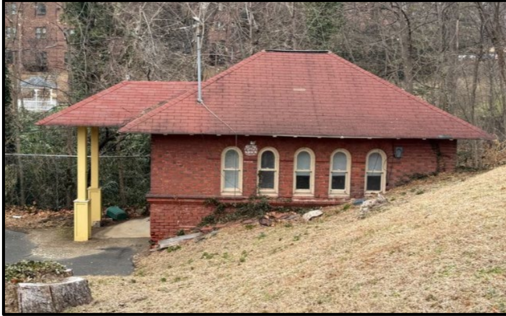
Figure 10. The south elevation of the stable. Source: Keeping Society of Philadelphia, 2026.
