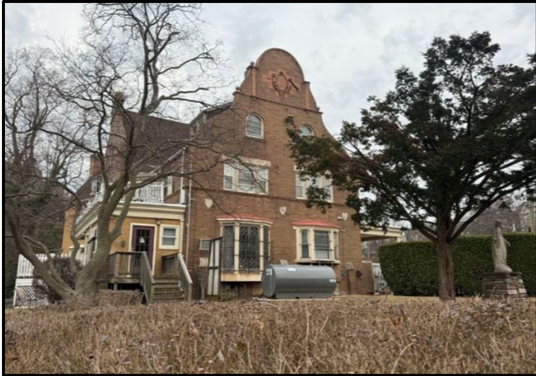
Figure 3. The south elevation. Source: Keeping Society of Philadelphia, 2026.
