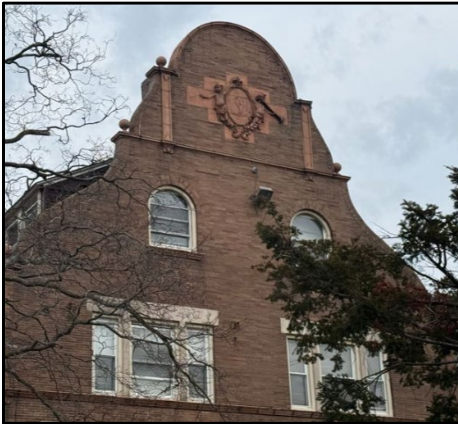
Figure 4. The upper portion of the Flemish gable in the primary (south) elevation. Source: Keeping Society of Philadelphia, 2026.
