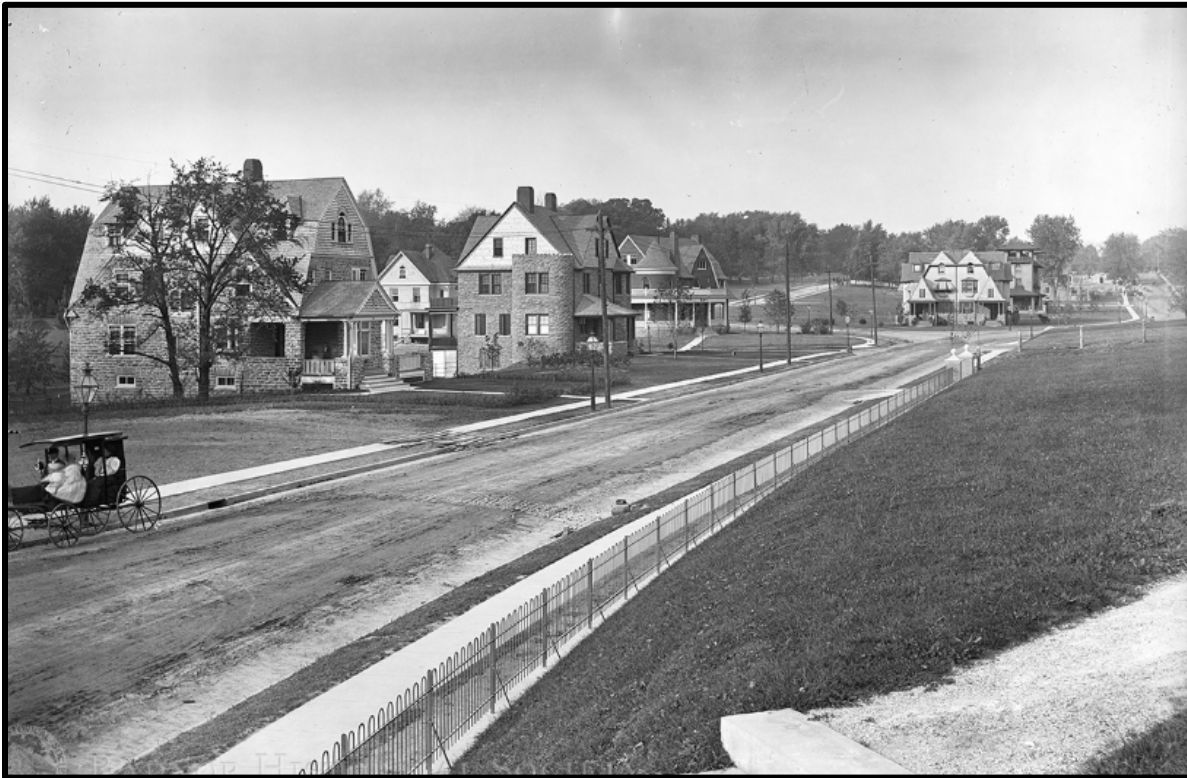
Figure 20. A view of Pelham Road in 1895. Source: Radnor Historical Society.
