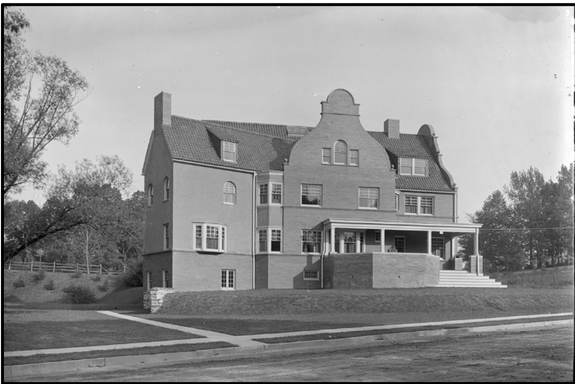
Figure 23. The primary (south) and east elevations of the subject building in 1895. Source: Radnor Historical Society.
