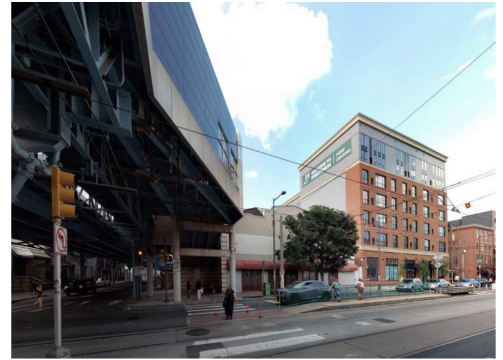
3 NORTHEAST VIEW FROM W. GIRARD AVE.
