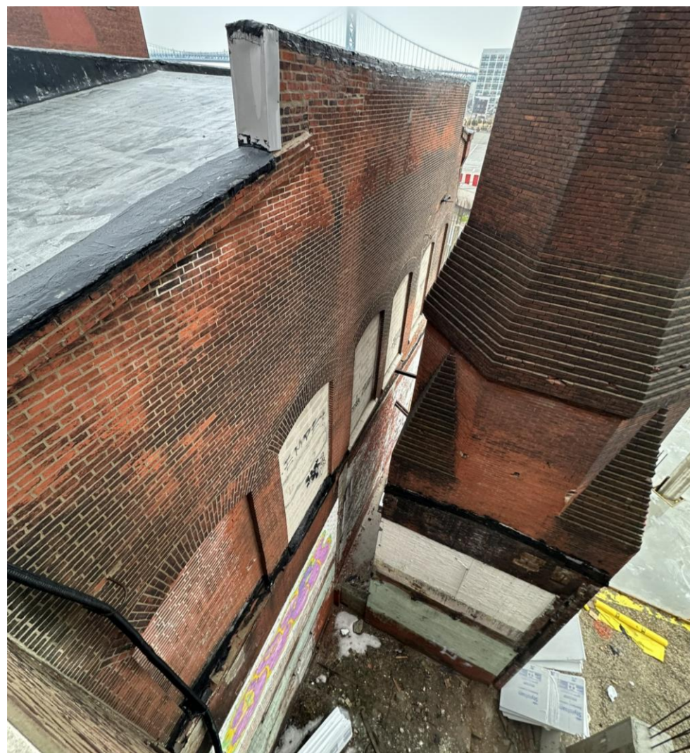
D - View looking South from Unit D roof
