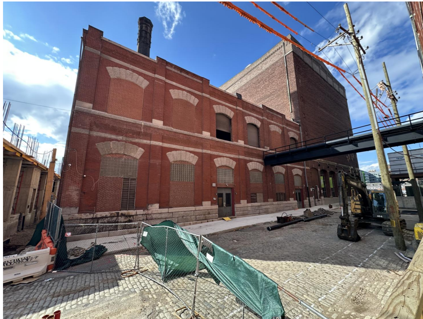
A - View looking West from decommissioned N Beach St
