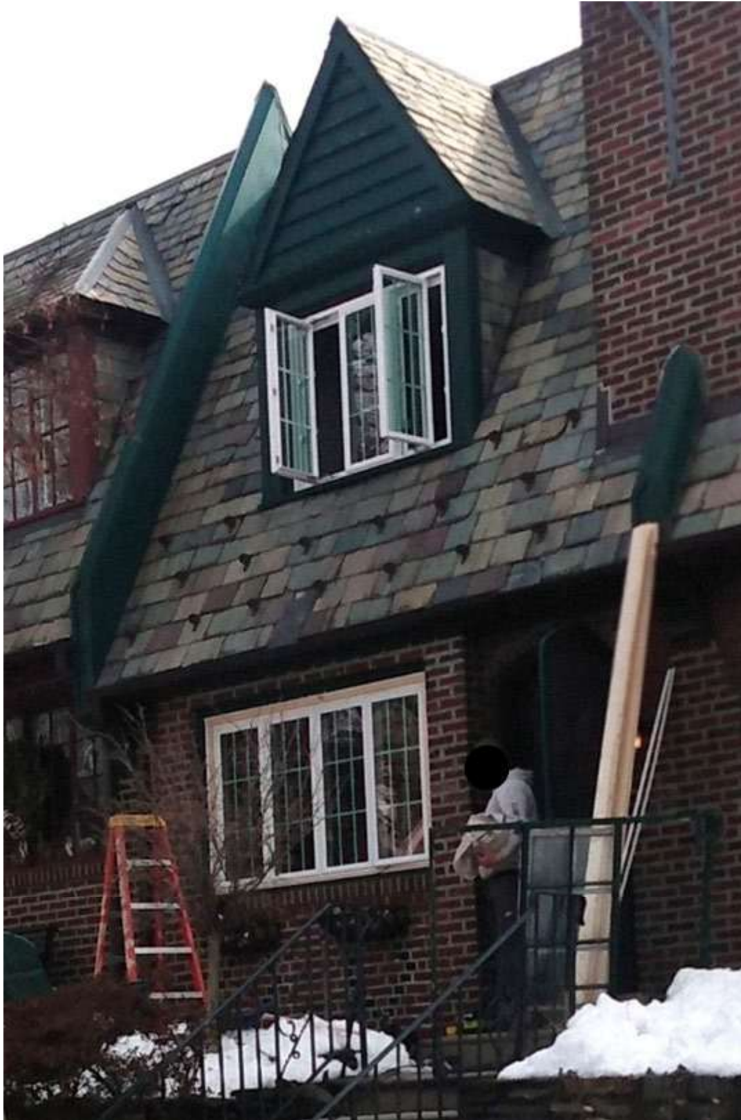
Image 2: 3440 W. Penn Street, showing new windows, February 2026.
