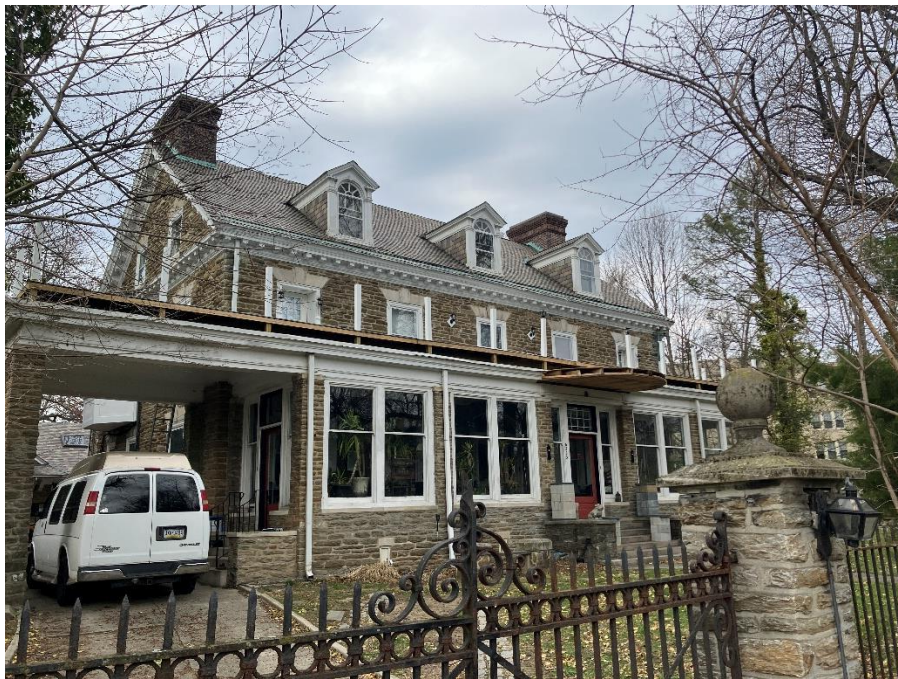
Image 2: 6363 Overbrook Ave, showing extent of work completed, on 3/30/2026.
