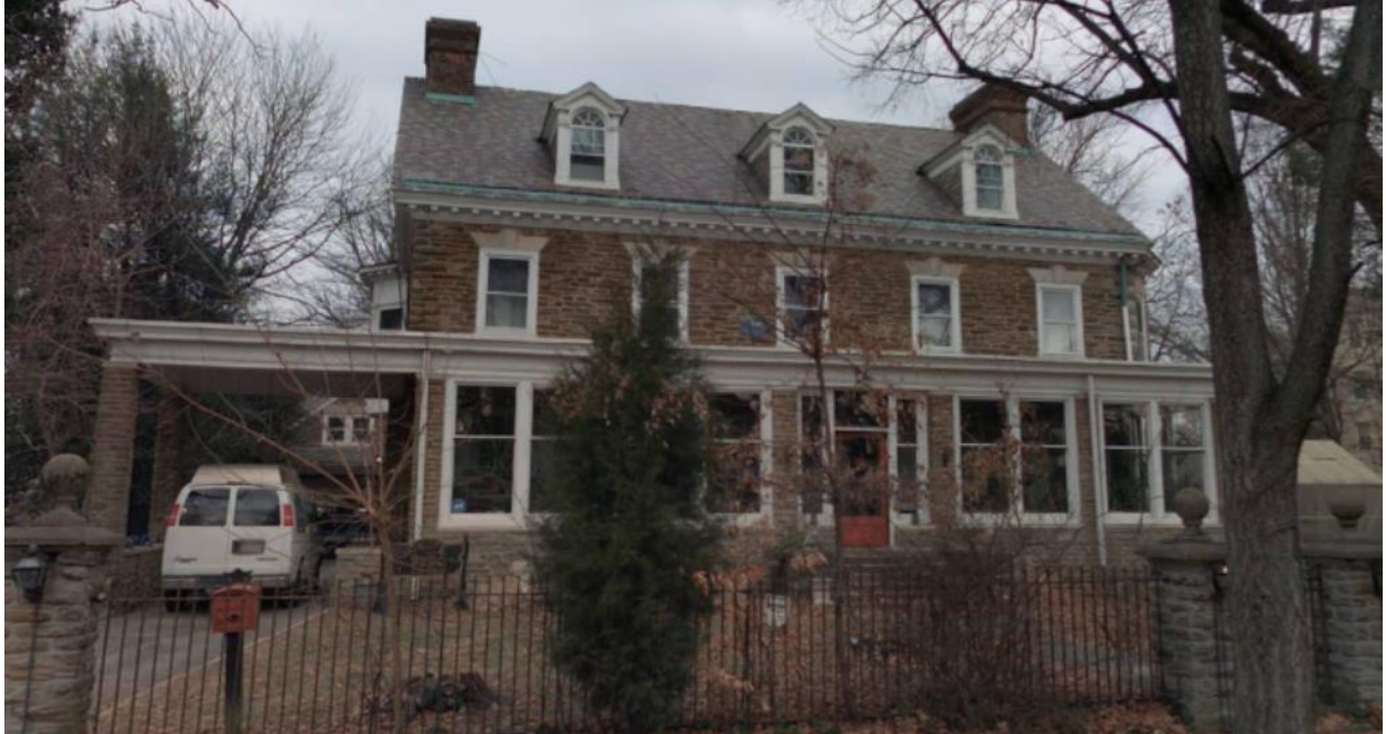
Image 1: 6363 Overbrook Ave, showing appearance before work was started. Cyclomedia, December 2022.
