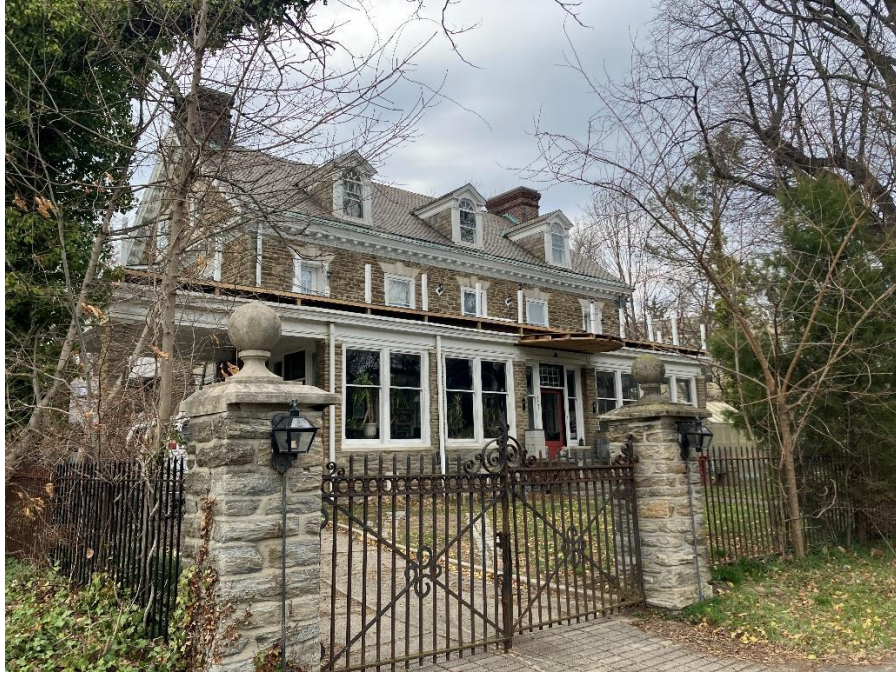
Image 3: 6363 Overbrook Ave, showing extent of work completed, on 3/30/2026.
