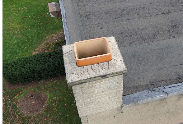
Replace brick wash coat
