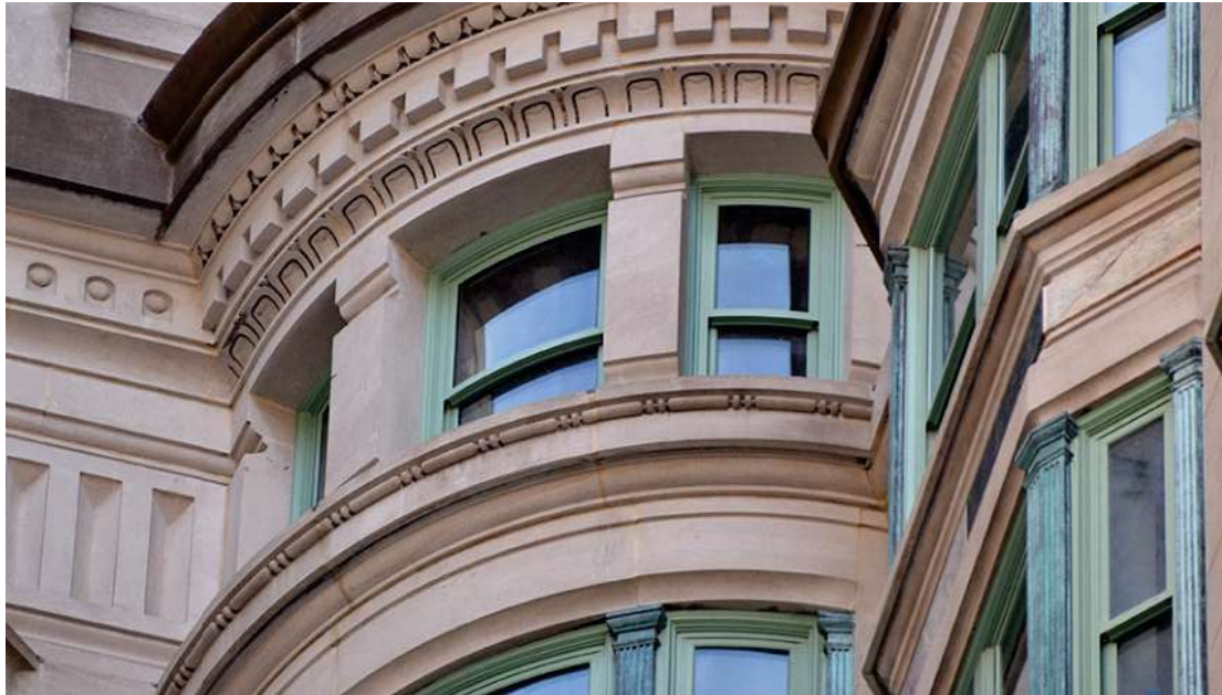
Mansion Windows, similar to Graham S2200 Double Hung with custom trim to match historic profile TBD
