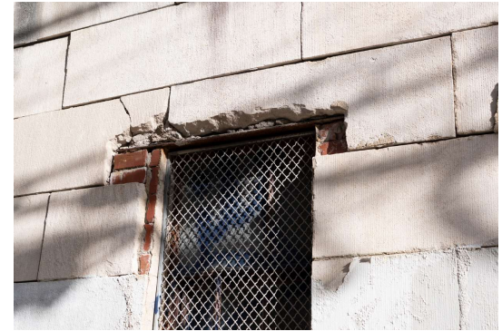
Replace damaged stone units
