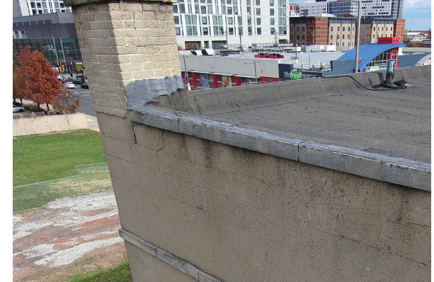
Repair detached stucco
