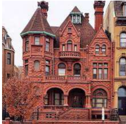
Ellis House, 1430 N Broad Street
