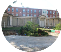
Conservatory (1909) Simon and Bassett 1 Story 3,150 GSF
