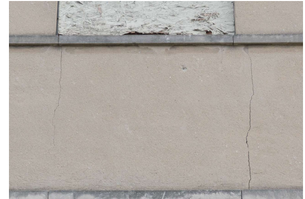
Repair stucco crack
