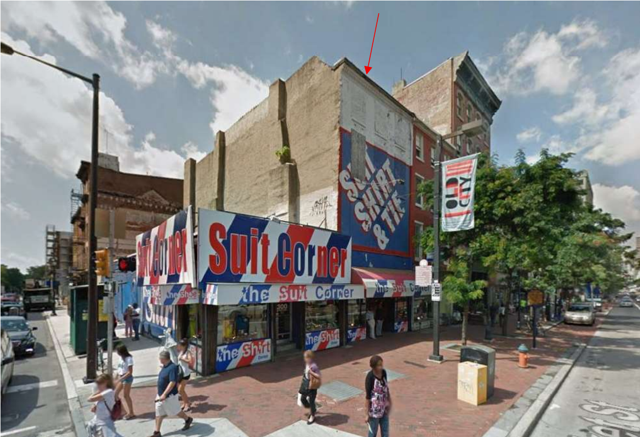
Figure 3: View from corner of 4 th and Market Streets, Aug 2013 (before fire):
