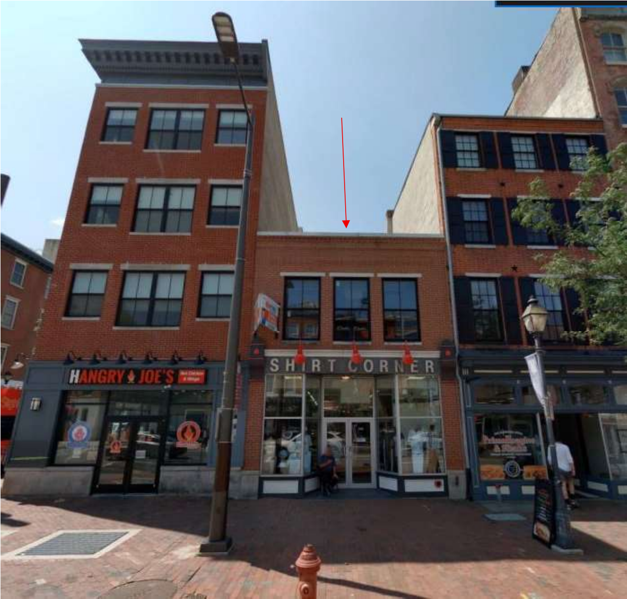
Figure 2: View of front façade of 302 Market St, July 2025:
