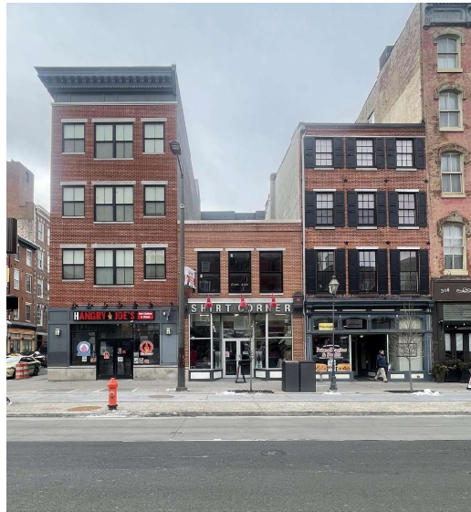
302 Market Street - Existing Condition
