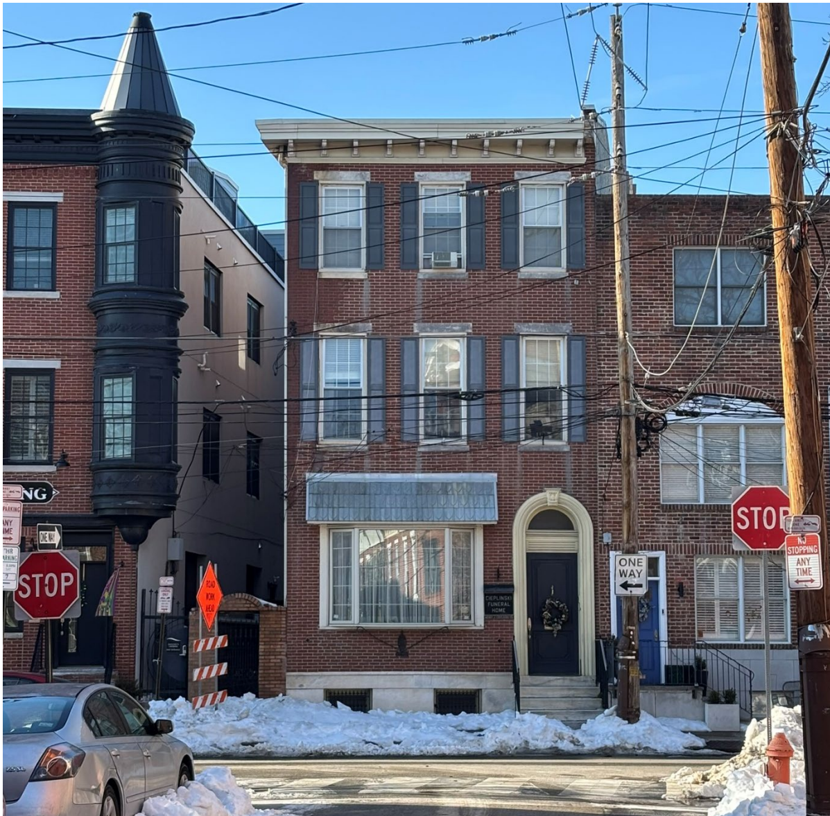
Figure 3. Photograph of 1018 S. 2nd Street front facade. Photograph by author, February 4, 2026.
