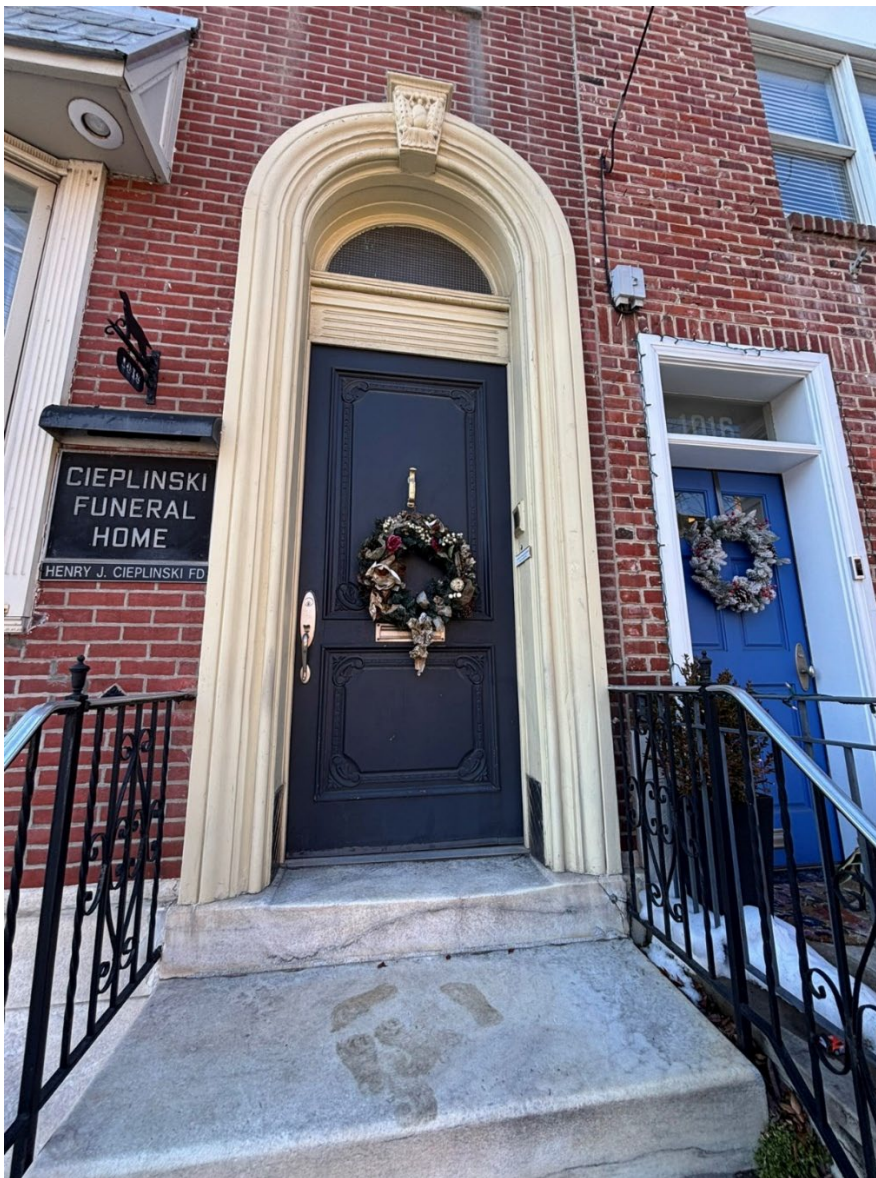
Figure 5. Main entrance at 1018 S. 2 nd Street, photograph by author, February 2026.
