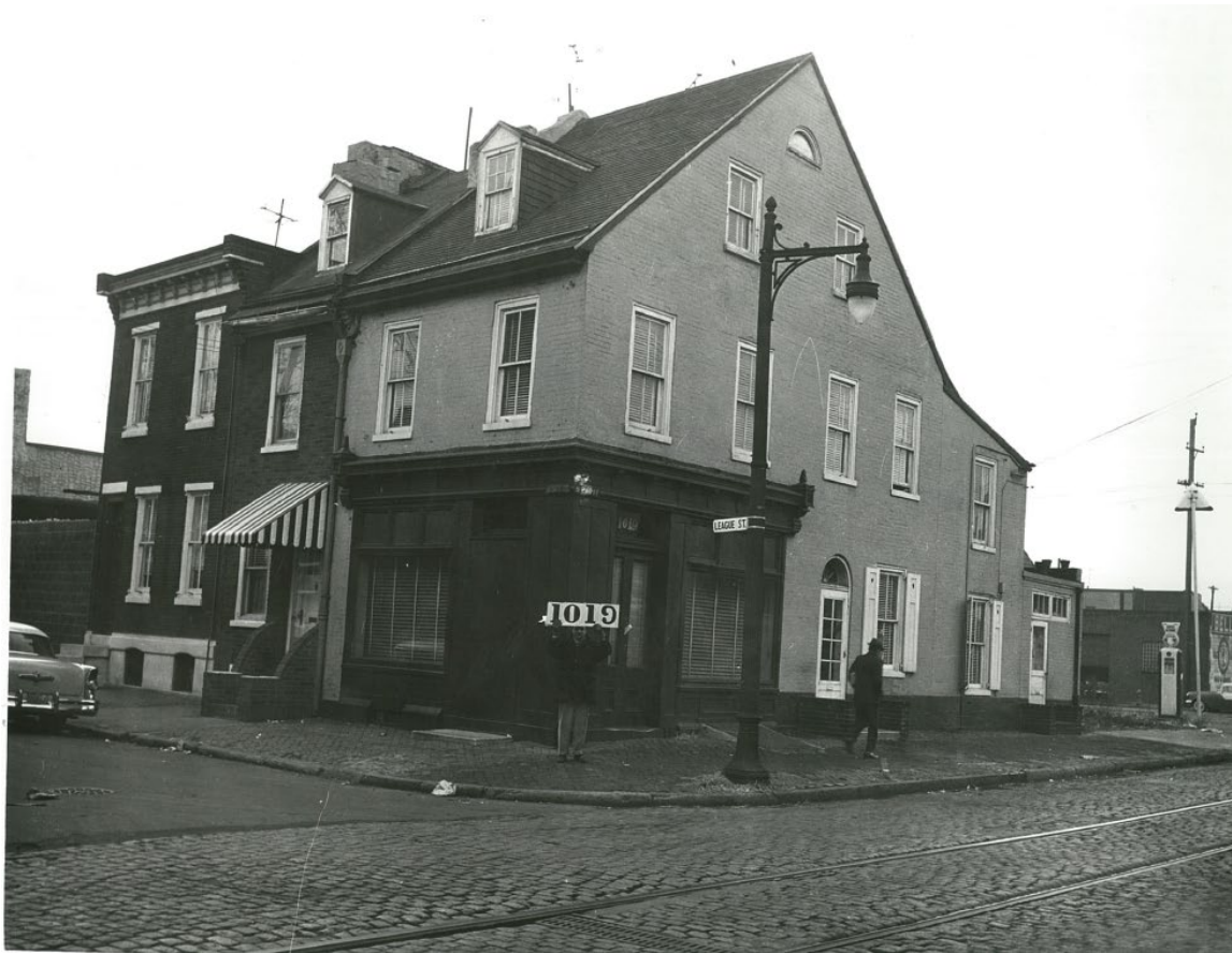
Figure 16. 1019 S. 2nd Street, now known as 144 League Street, directly across the street from the subject property. This photograph is from 1957, shortly before the storefront was removed and the first floor restored to a residential appearance. This was the building which housed the Nebinger brothers' apothecary for many years. Source: Philadelphia Historical Commission archive.
