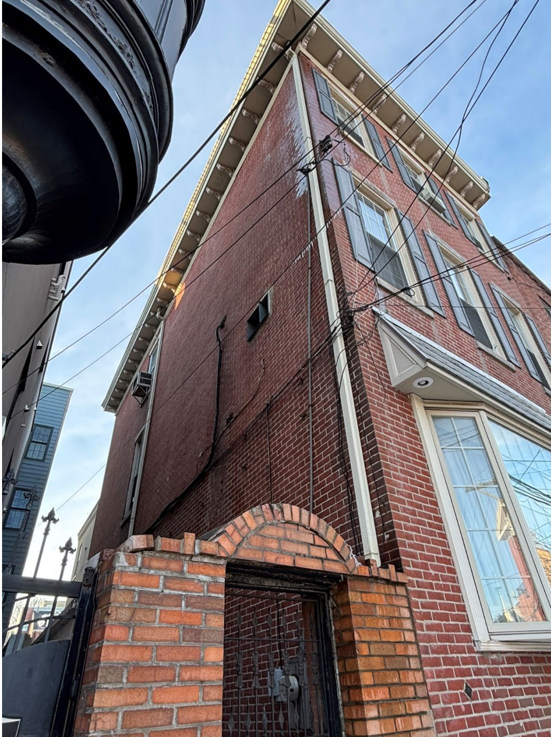
Figure 7. South facade (left side) of the building featuring red brick, a mechanical vent, electrical conduit, and two windows towards the rear. Photograph by author, February 2026.
