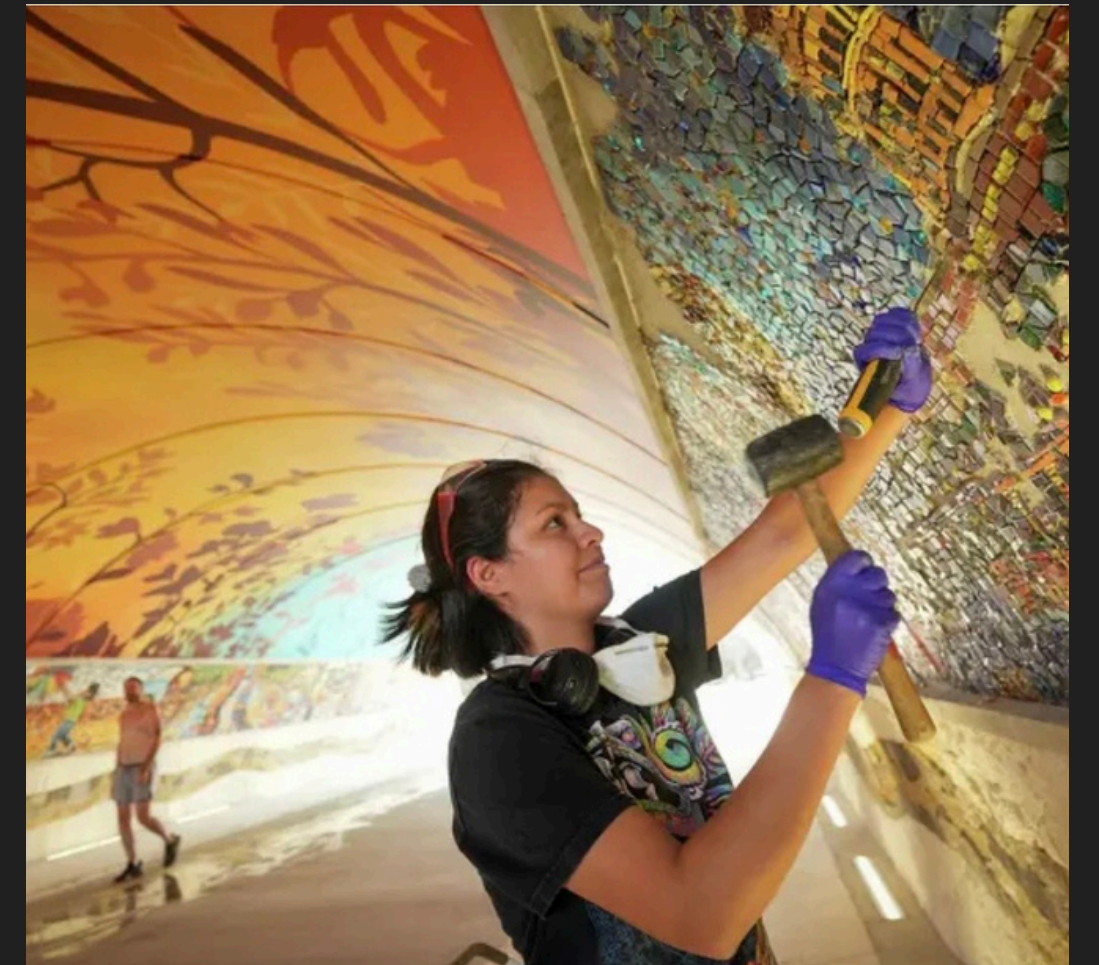
Glass & Porcelain Tile Mosaic Installation
