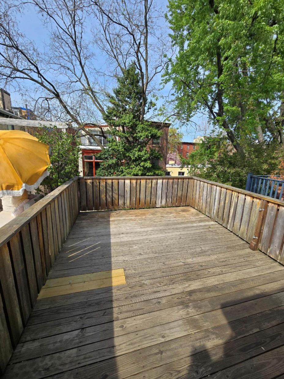
Looking north from existing 2027 deck 5/5/25
