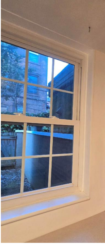
2029 rear window showing masonry jamb depth
