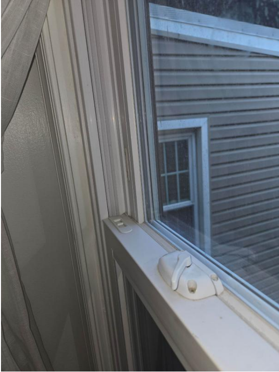
2027 rear window showing 2x4 Frame jamb depth
