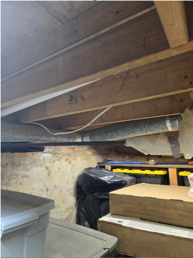
Addition Framed into alley at 2027. Wood Frame over slab on grade.
